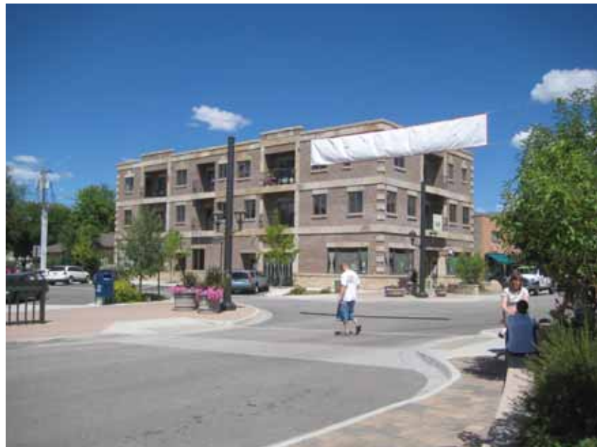
CONCRETE CROSSWALK WITH BULB-OUTS
