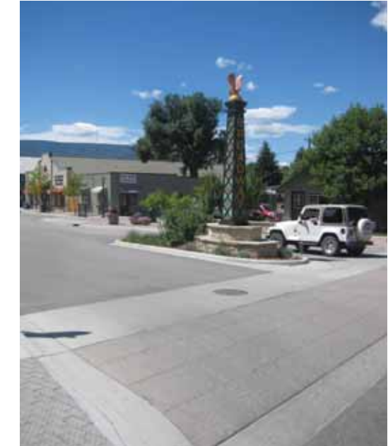
RAISED CONCRETE CROSSWALK
