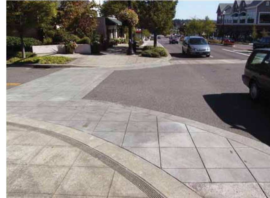
FLUSH CONCRETE BULB-OUT & CROSSWALK
