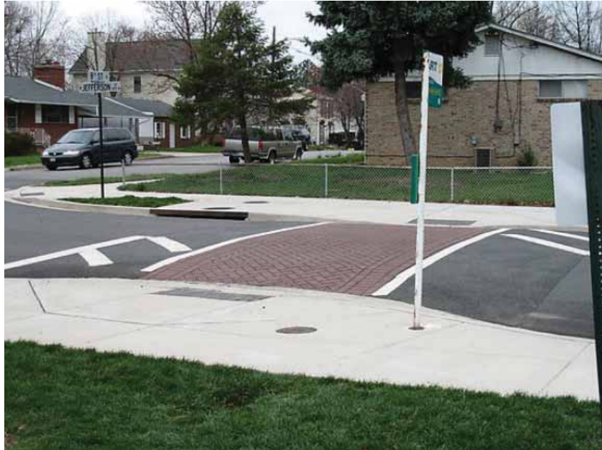
RAISED CROSSWALK WITH STAMPED CONCRETE
