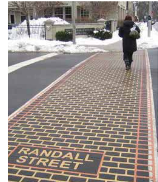
PAINTED PATTERN IN CROSSWALK
