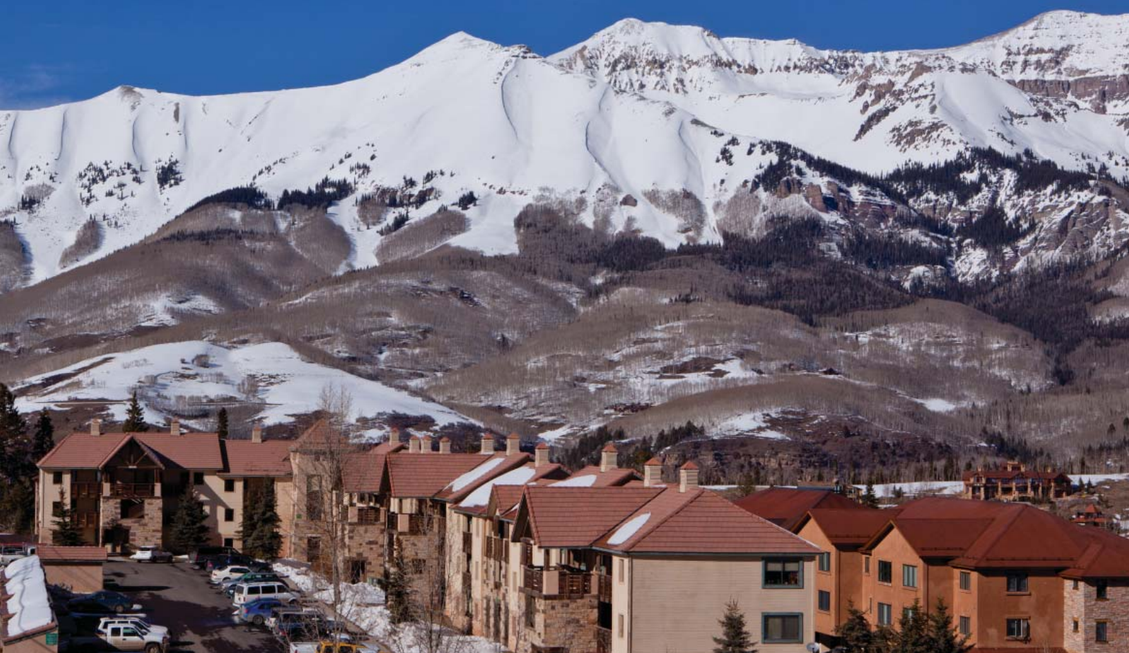
View toward VCA from parking garage
