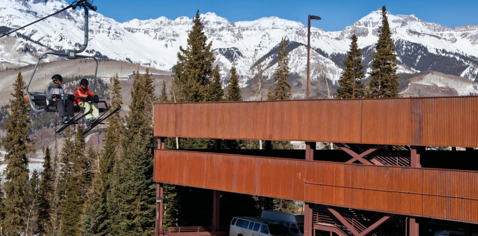
Parking garage existing conditions
