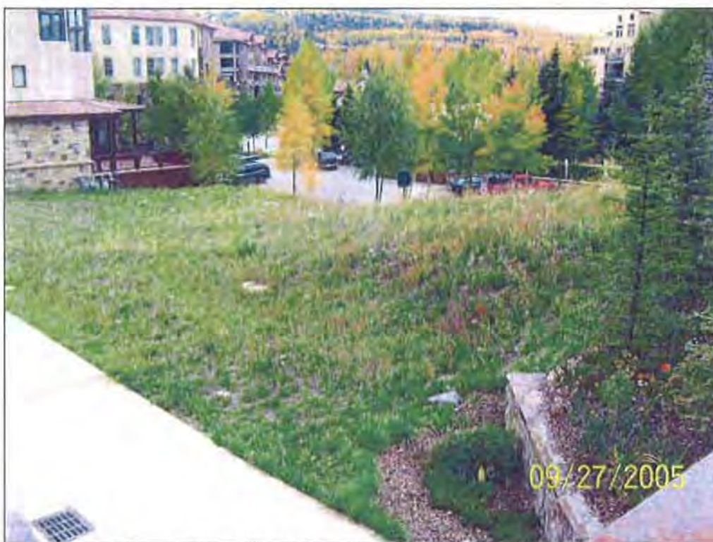
Looking southwest across the lots from the Mountain Village Boulevard overpass, the Shirana Condominiums (far upper left) and the western parking lot can be seen. The Wyndham Peaks can be seen in the far upper right.
