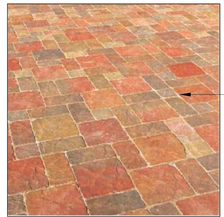
2 Concrete Unit Pavers Type II SCALE: 1/2" = 1'-0"
