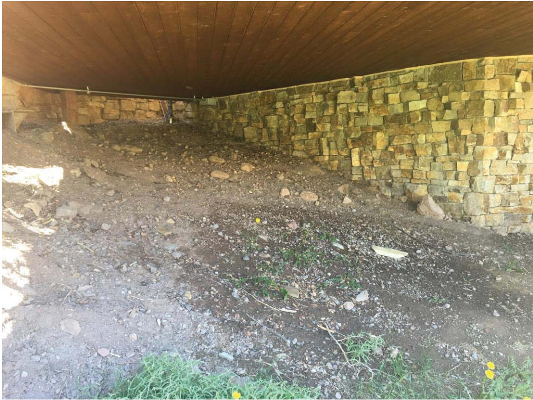
Area Under Unit A101 Deck
