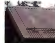
CORRUGATED METAL ROOF
