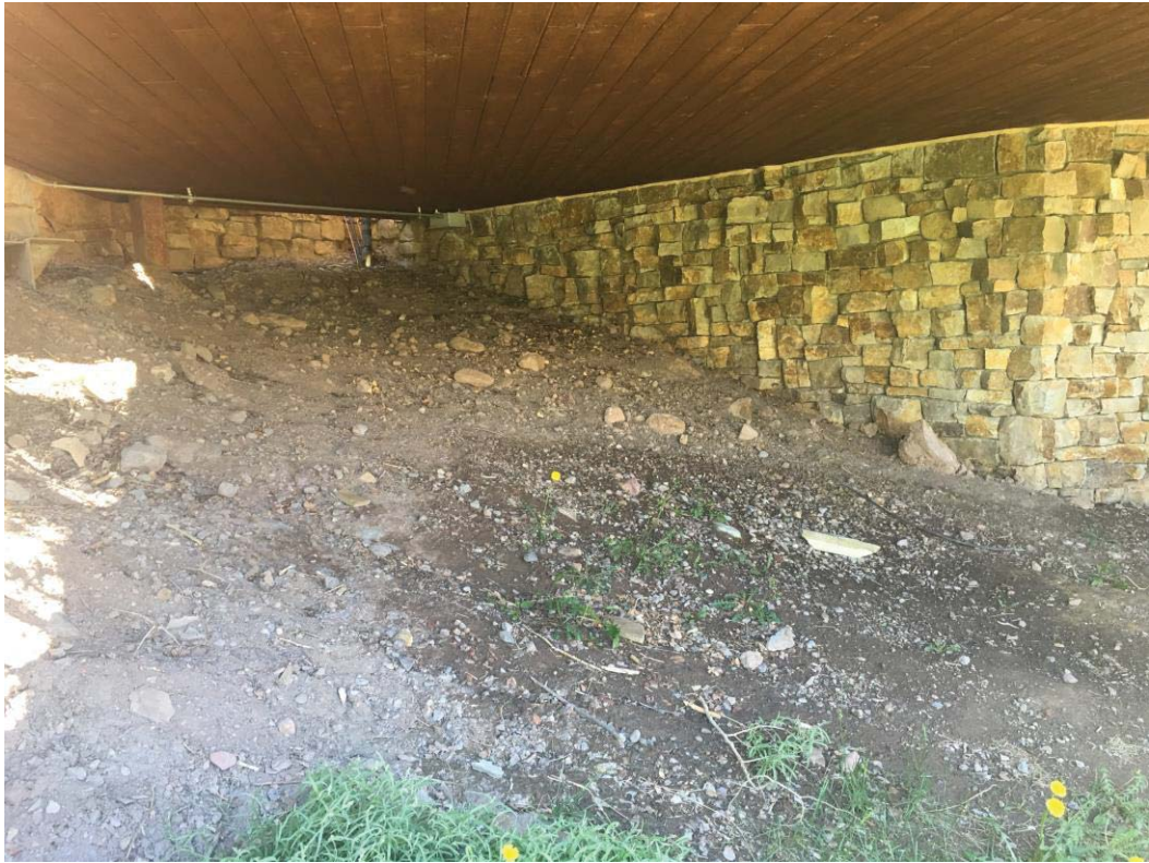
Area Under Unit A101 Deck
