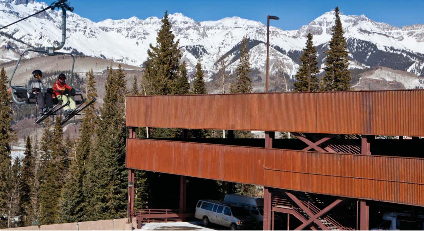
Parking garage existing conditions
