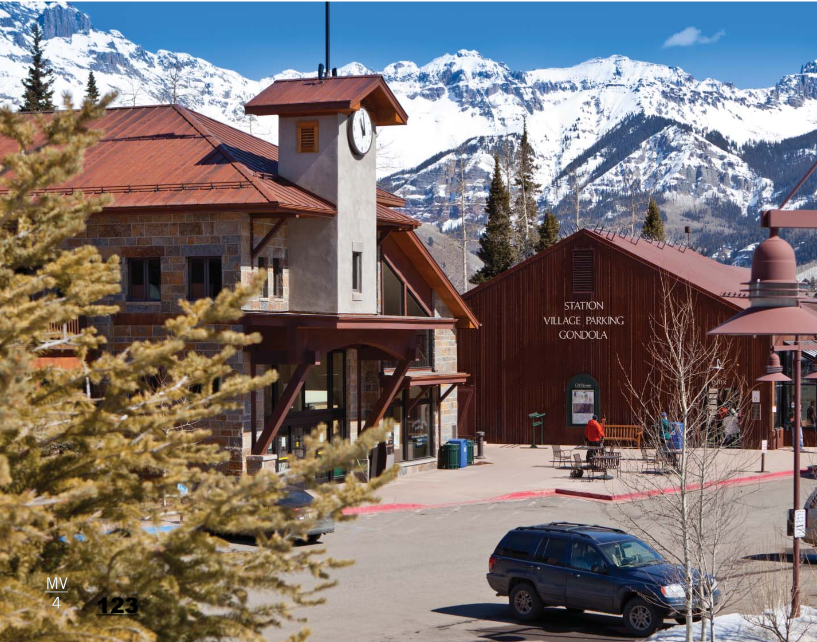
Town Hall Center Subarea existing conditions
