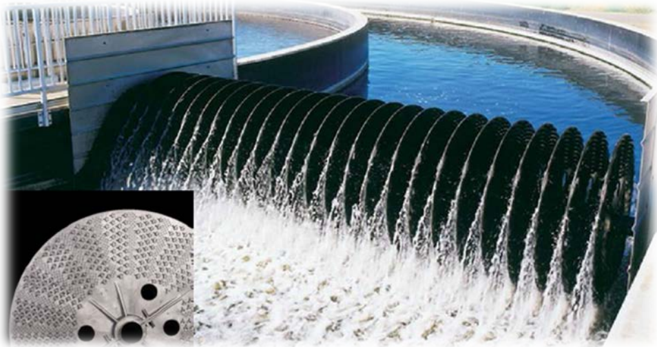
Expand Existing Aeration System
