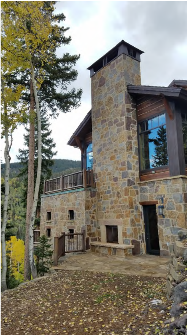
EXISTING PATIO IN 30' GENERAL EASEMENT
