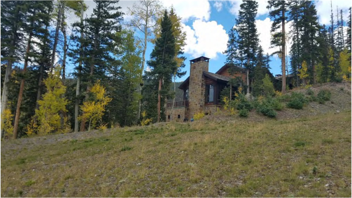
EXISTING SITE PHOTO
