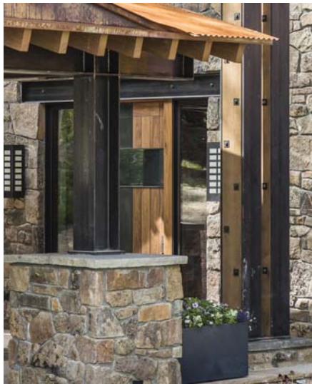
Structural steel elements and banding
