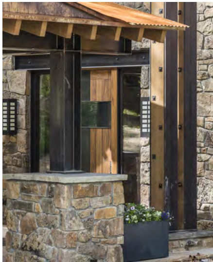
Structural steel elements and banding
