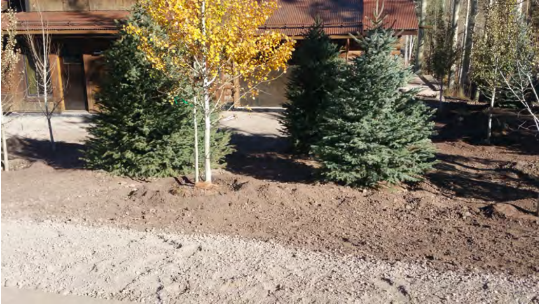
Sidewalk approved in 2014 does not work with grades and access to street from this view
