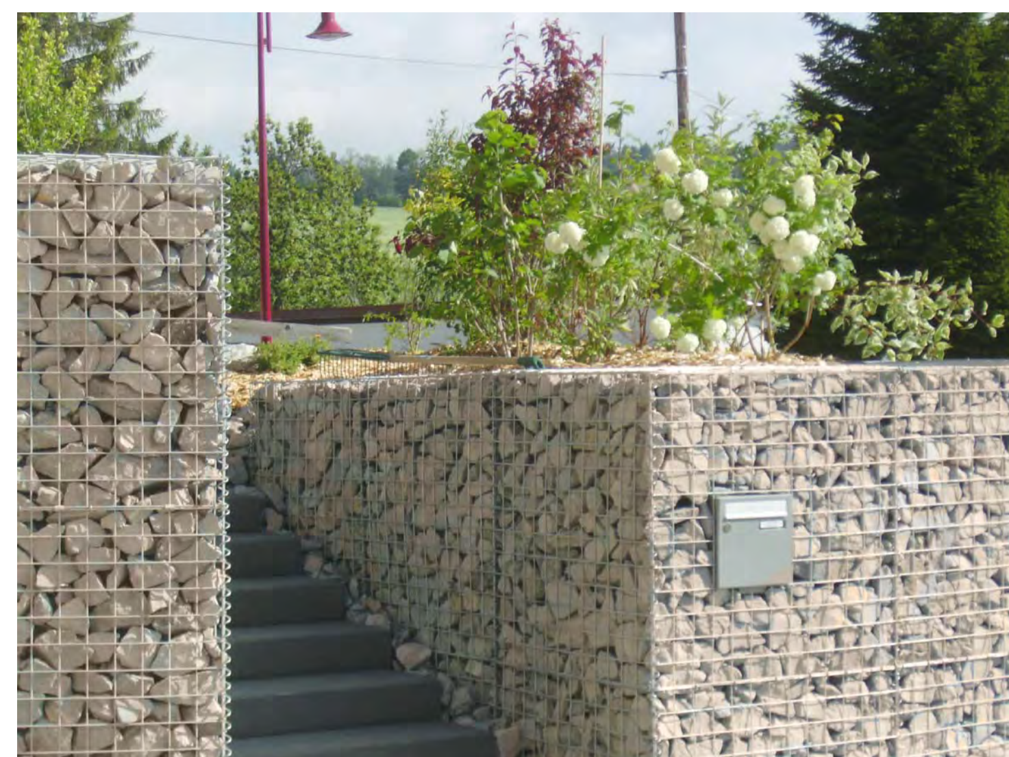
7 RUBBLE STONE IN HILFICKER WALL/ LWR. RETAINING SCALE: NO SCALE
