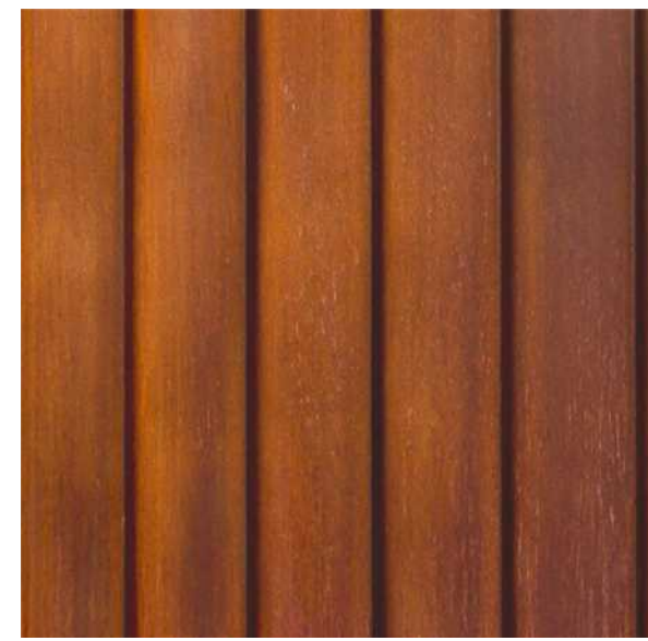
R1 STANDING SEAM ROOF RUSTED
