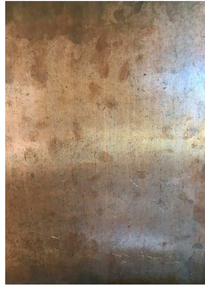
W3- 24" VERTICAL COPPER PANEL SIDING / FASCIA
