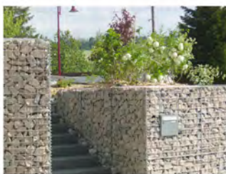
7 RUBBLE STONE IN HILFICKER WALL/ LWR. RETAINING SCALE: NO SCALE
