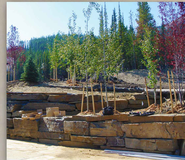
TERRACED BOULDER RETAINING WALLS
