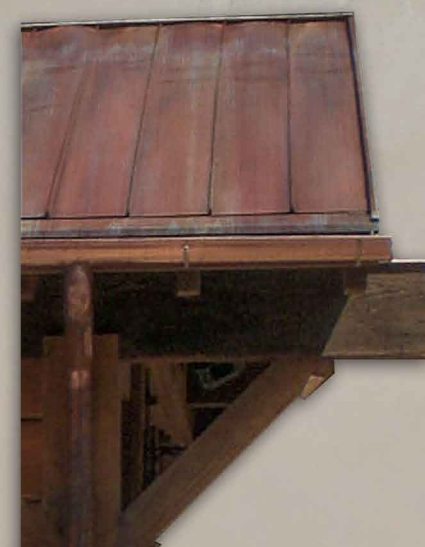
STANDING SEAM CORTEN ROOFING
