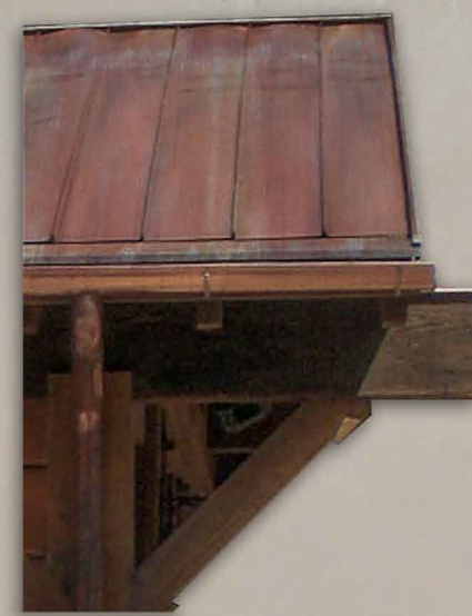
STANDING SEAM CORTEN ROOFING
