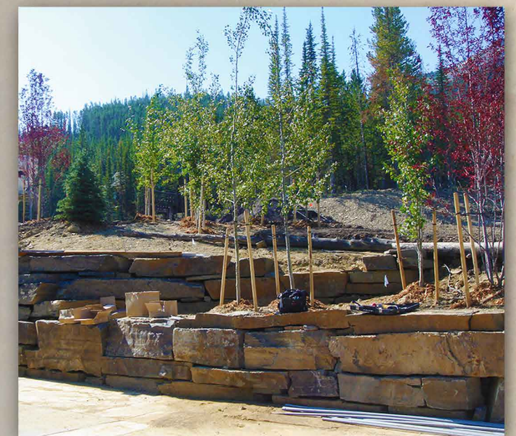
TERRACED BOULDER RETAINING WALLS
