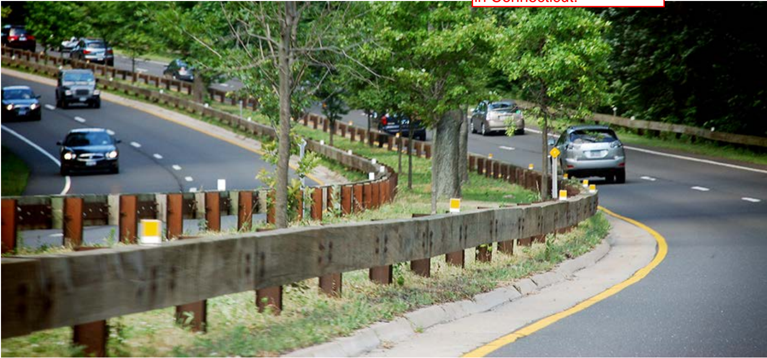
Guardrail Image- Reference Merritt Parkway in Connecticut.
