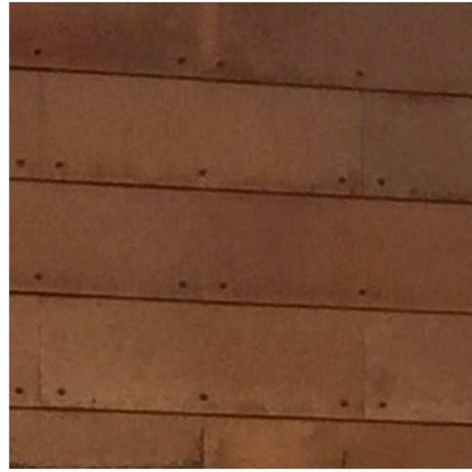
RUSTY METAL PANEL
