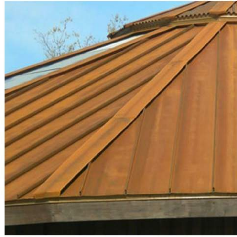
STANDING SEAM METAL ROOF
