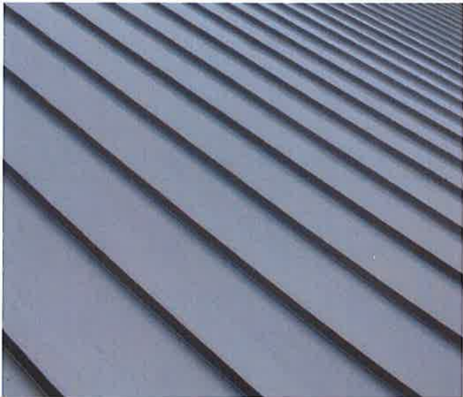
STANDING SEAM ROOF
