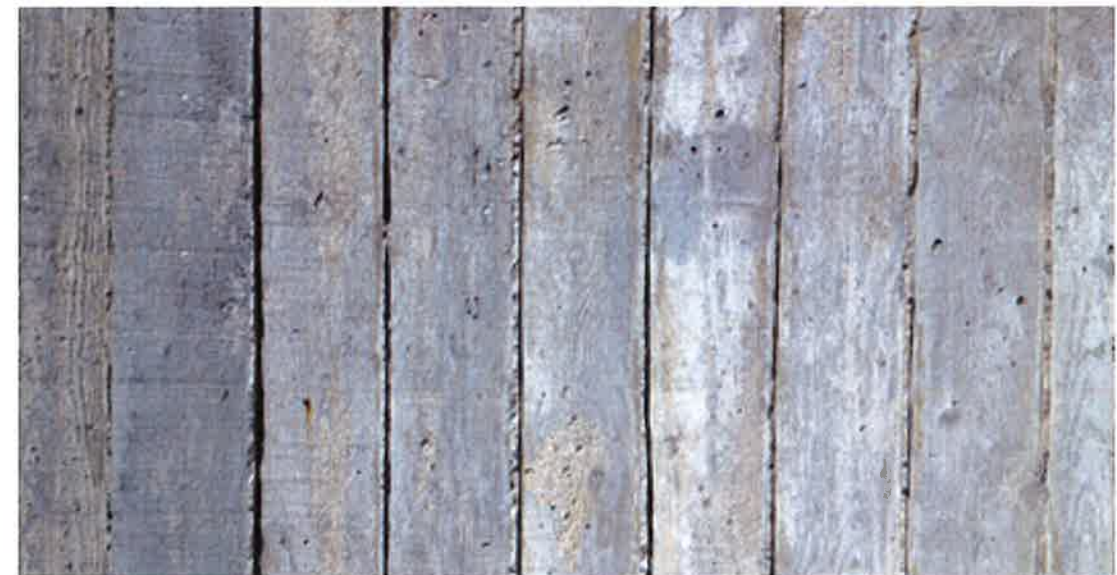
BOARD FORMED CONCRETE
