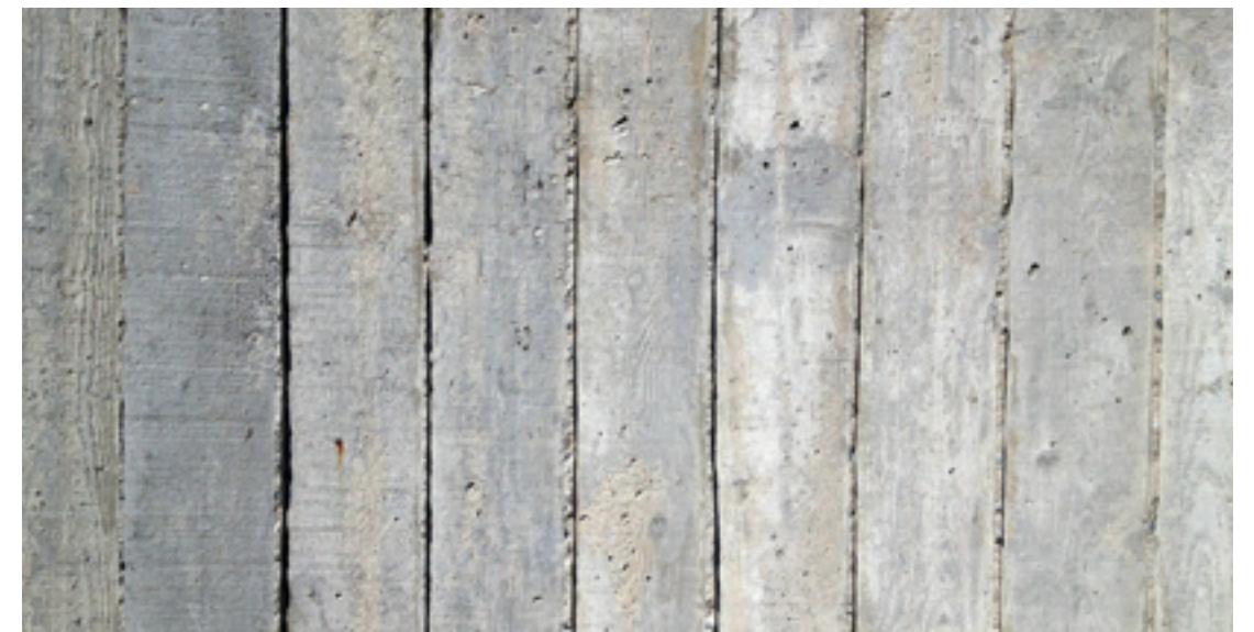
BOARD FORMED CONCRETE
