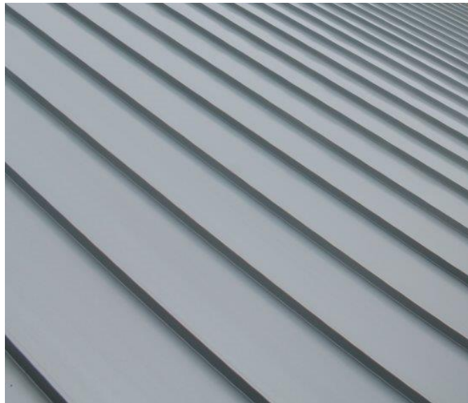
STANDING SEAM ROOF
