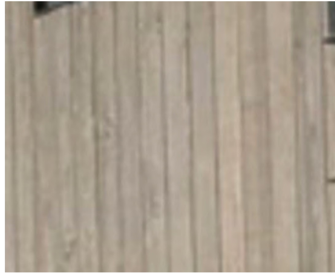
1 OPTION A - VERTICAL CEDAR 1x6 CEDAR W/ 1/4" REVEAL, SHIPLAP, GRAYWASH STAIN, SEALED
