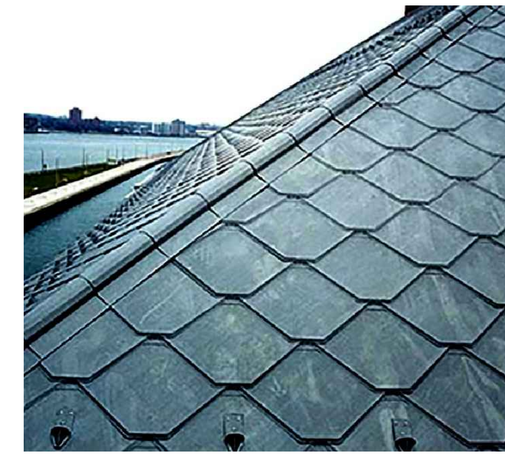
CASTLETOP METAL SHINGLES FINISH: WEATHERED ACRYLIC COATED GALVALUME MANUFACTURER: ATAS INTERNATIONAL
