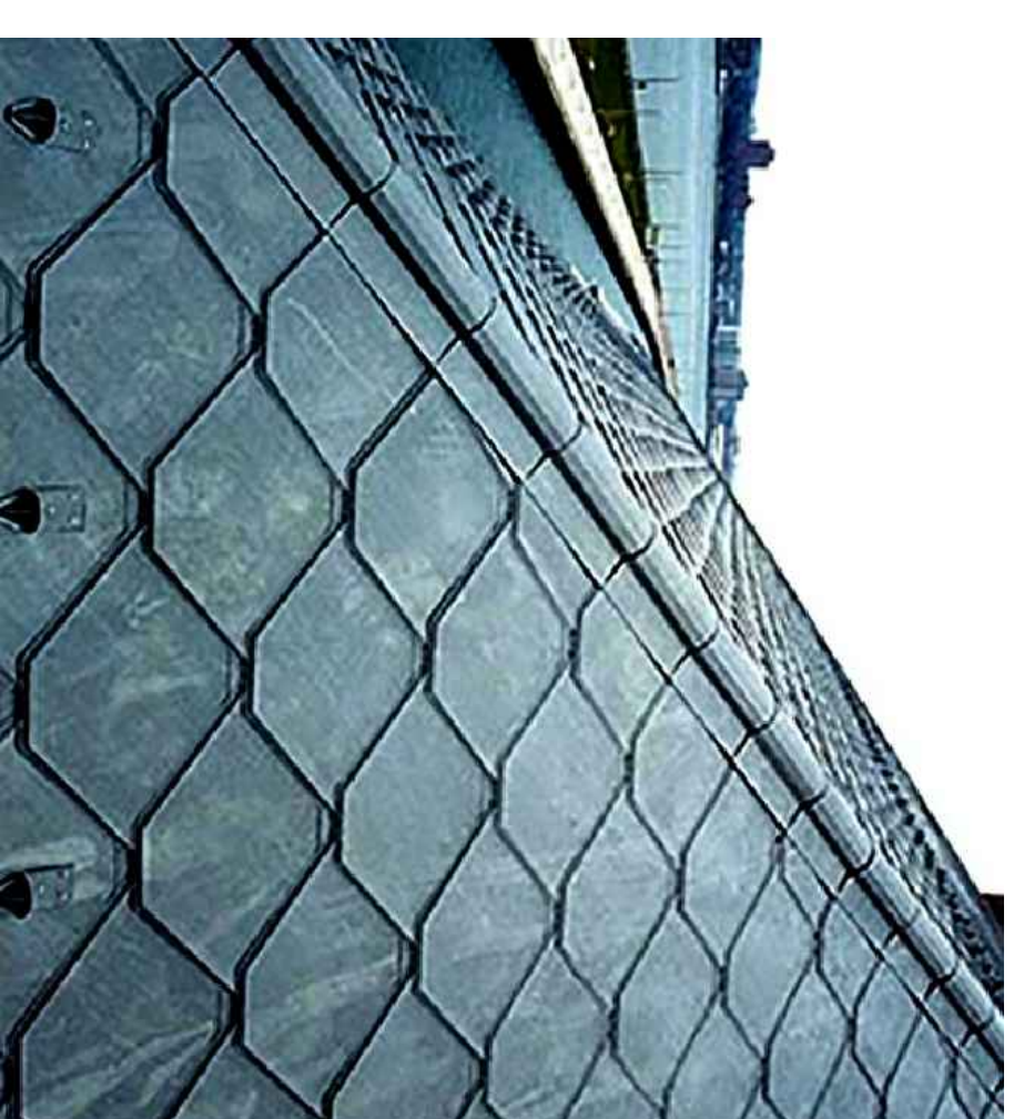
CASTLETOP METAL SHINGLES FINISH: WEATHERED ACRYLIC COATED GALVALUME MANUFACTURER: ATAS INTERNATIONAL
