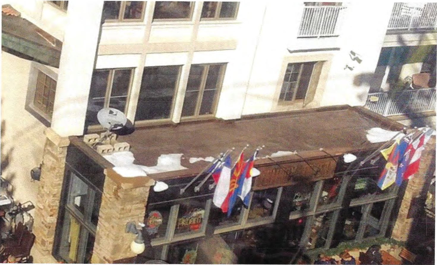
New roof brown membrane.
