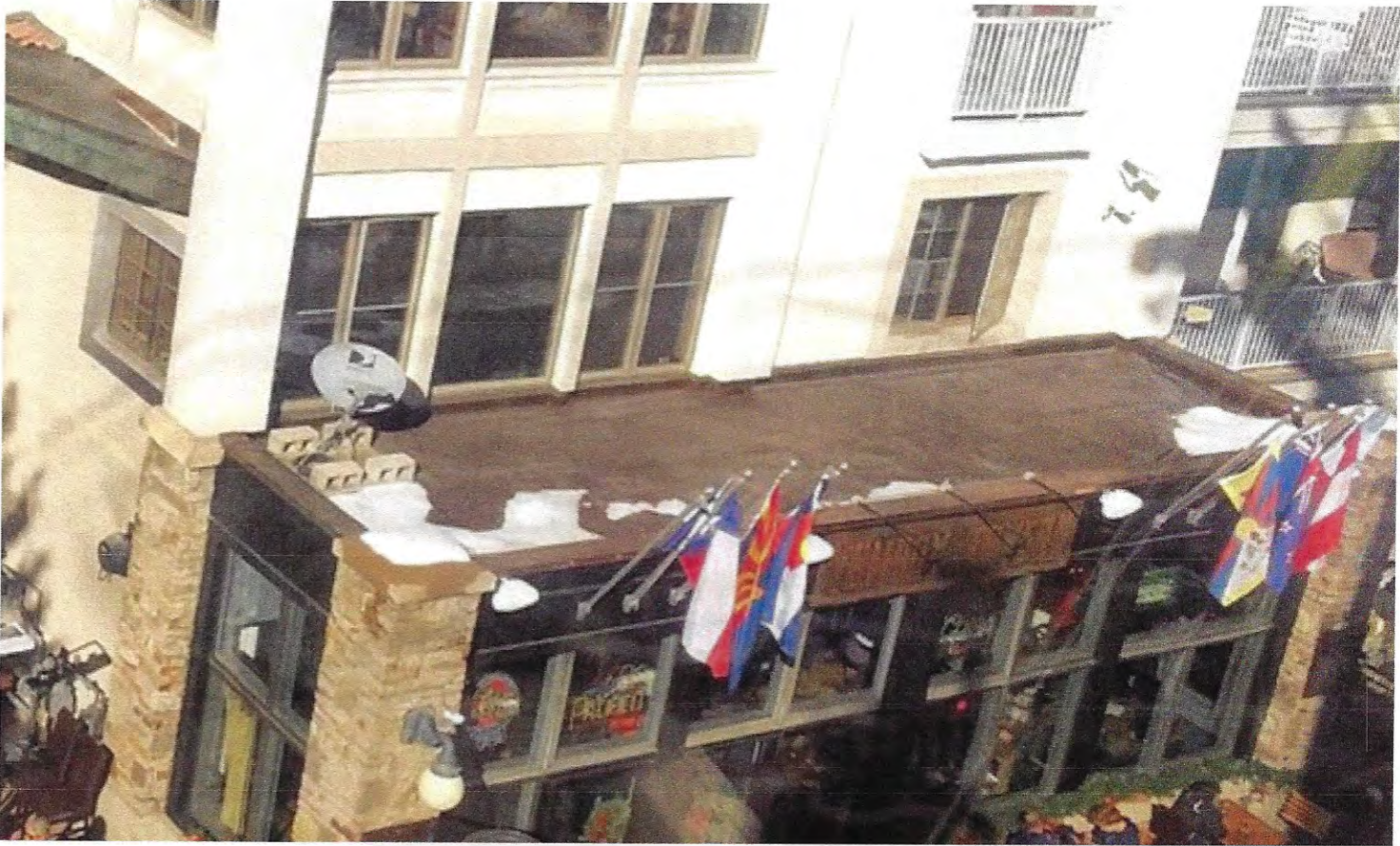
New roof brown membrane.
