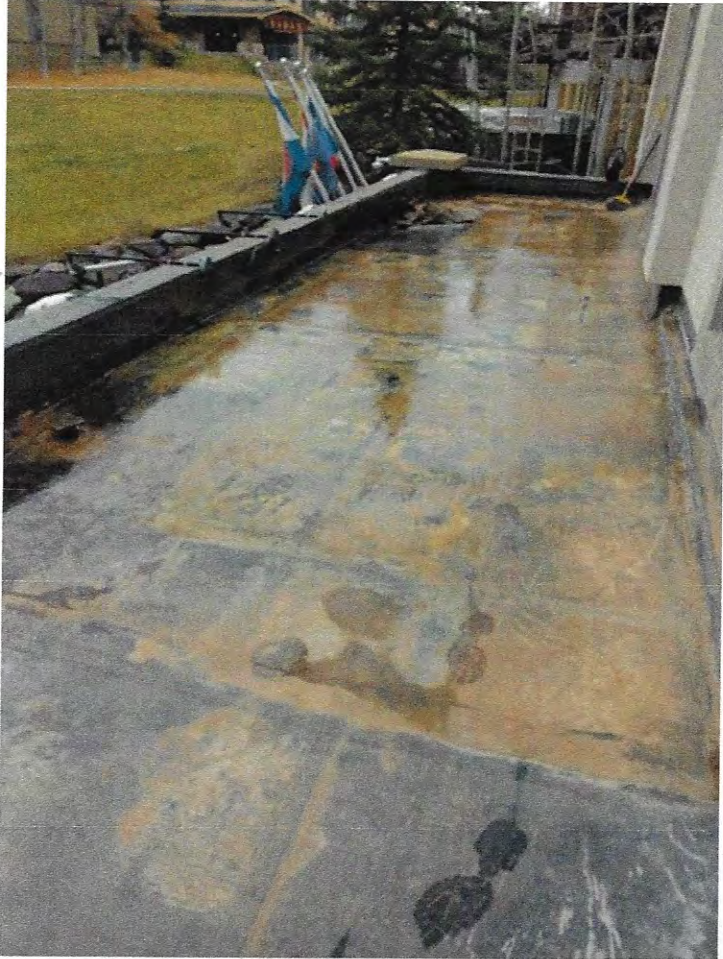
Roof without the tiles or IB membrane.
