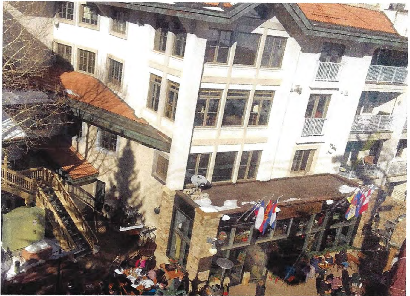
New roof with brown membrane.
