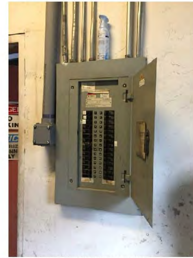
Photo #10: Existing Repair Garage panel
