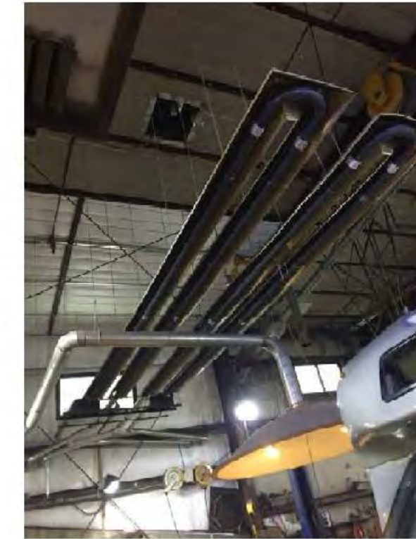
Photo #1: Radiant tub heaters in the Repair Garage
