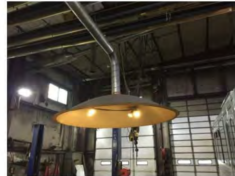
Photo #7: Repair Garage welding hood
