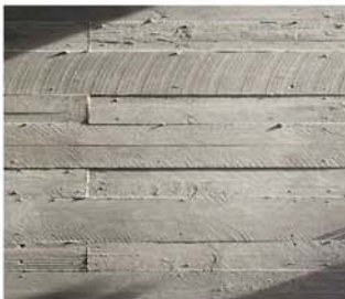
BOARD FORM CONCRETE
