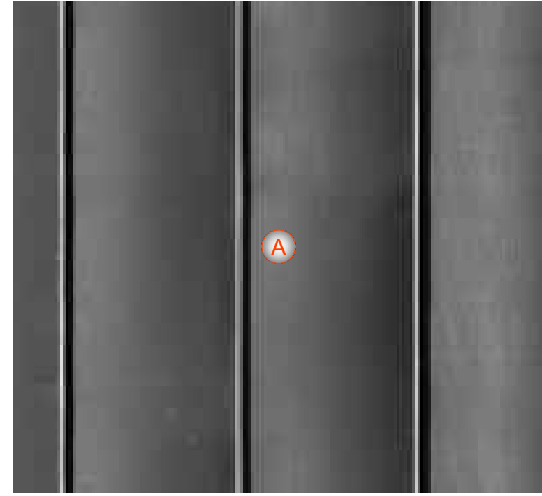
STANDING SEAM METAL ROOF
