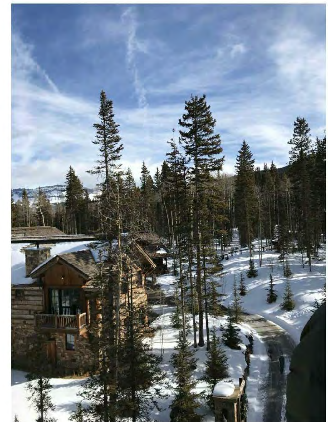
2 VIEW TO SOUTHWEST NEIGHBOR SCALE: NO SCALE
