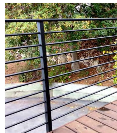
METAL RAILING, PAINTED BLACK
