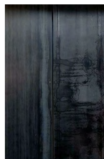
METAL SIDING, UNPAINTED MILL STEEL
