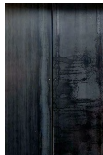
METAL SIDING, UNPAINTED MILL STEEL
