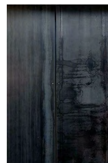
METAL SIDING, UNPAINTED MILL STEEL
