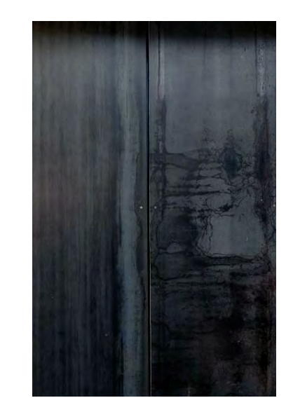
METAL SIDING, UNPAINTED MILL STEEL
