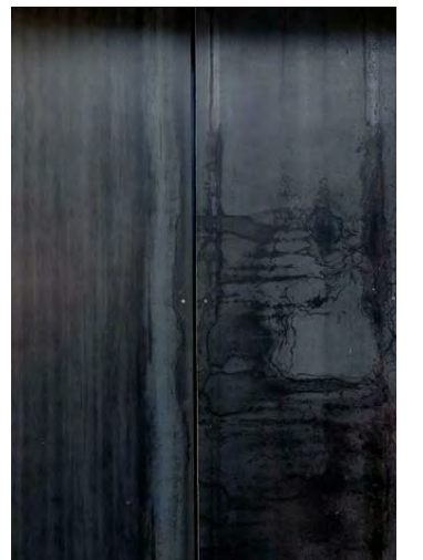
METAL SIDING, UNPAINTED MILL STEEL
