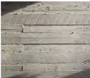
BOARD FORM CONCRETE
