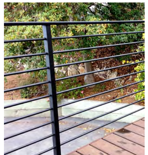
METAL RAILING, PAINTED BLACK
