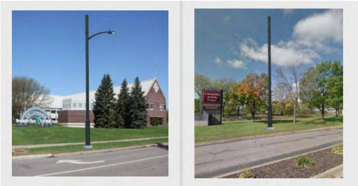
2) Small cell integrated within light pole
