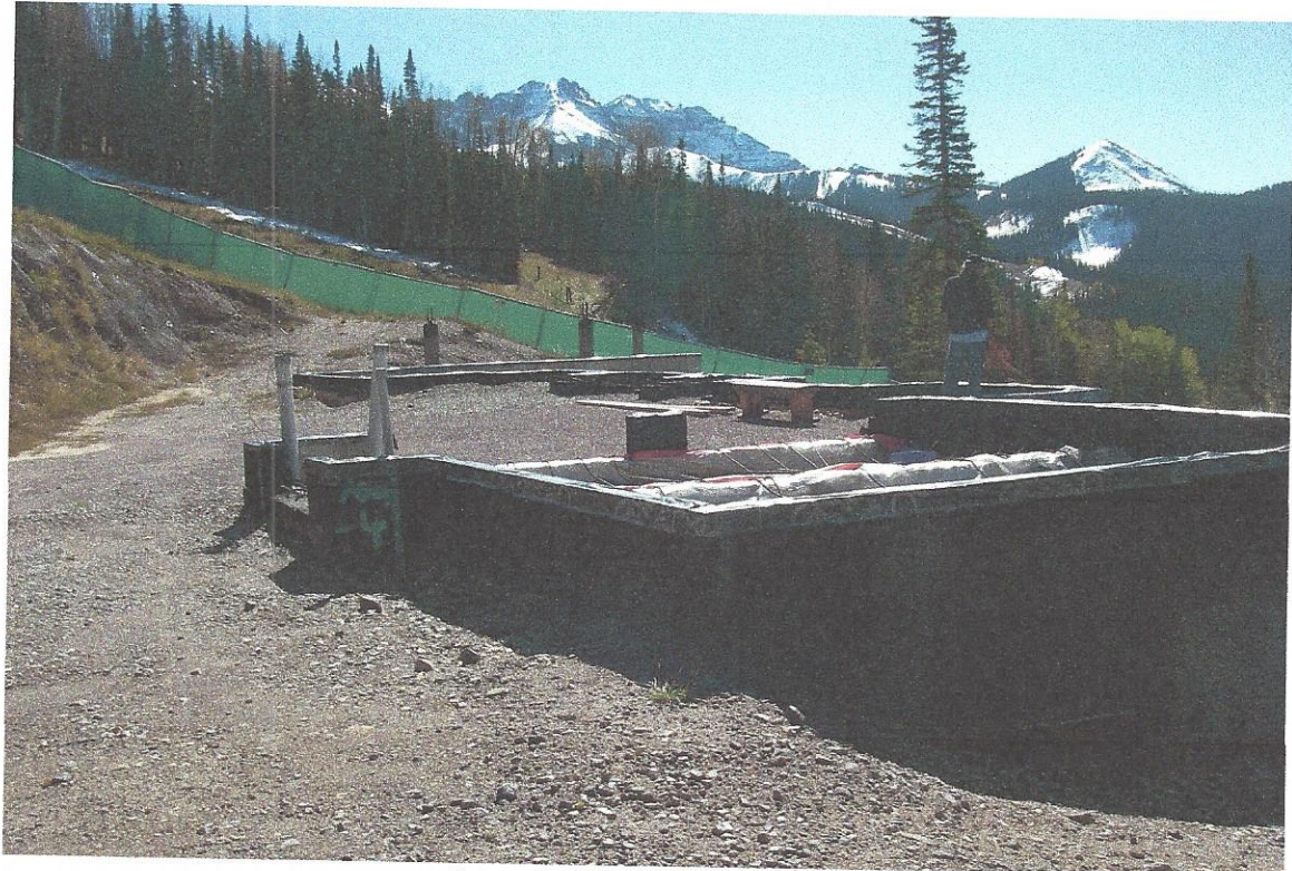
EXISTING FOUNDATION & AUTO COURT
