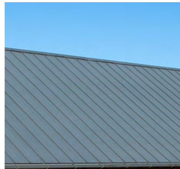
Roofing / (Drip Edge) - Standing Seam 16" O.C.
