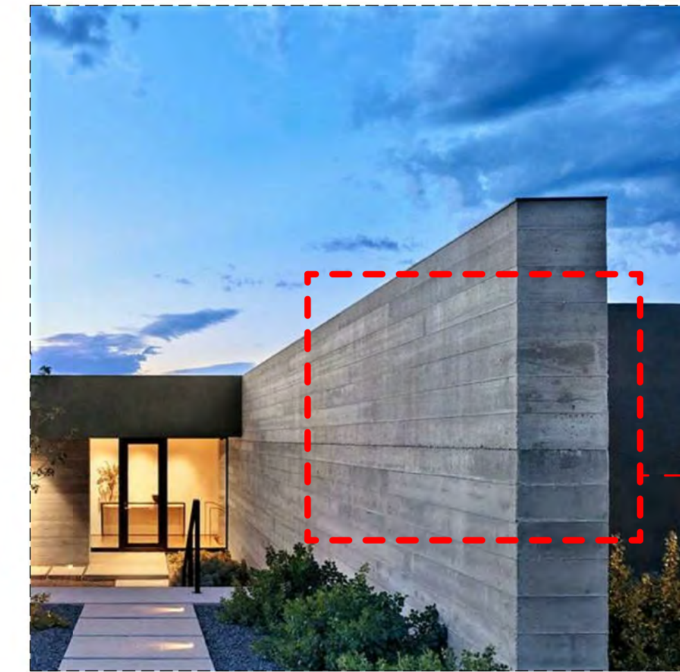
BOARD FORMED CONCRETE
