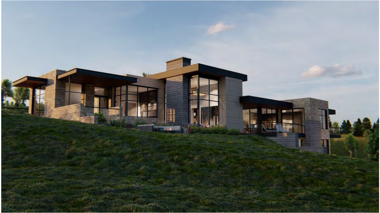
Fig. 4 – From Pennington Place. Retaining walls on the east side of both the pool and hot tub keep them hidden from public view.
