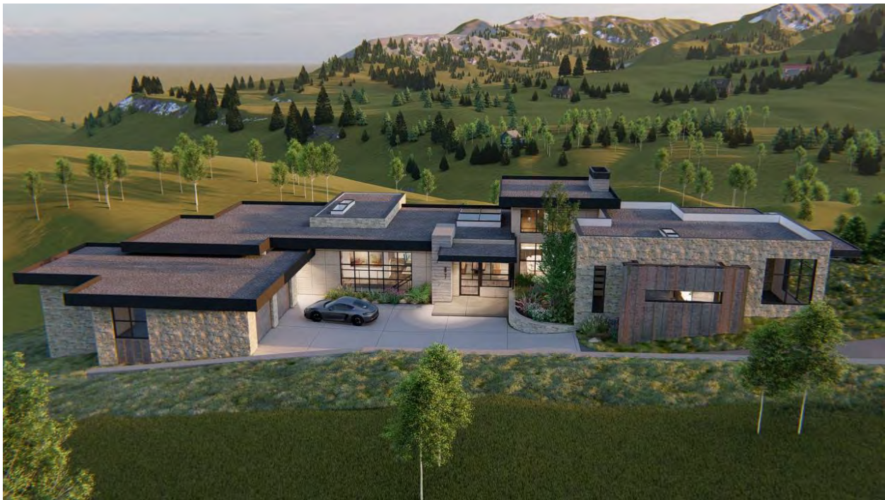
Fig. 1 – Note how the flat roofs must “step down” with the grade to keep under the Private Restrictive Covenant Agreement.
