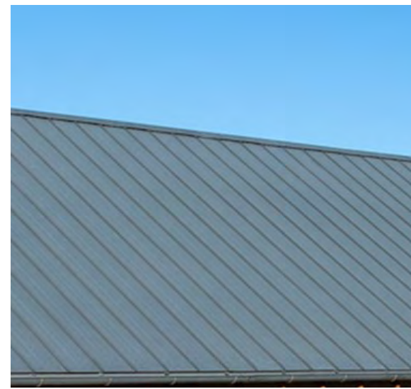
Roofing / (Drip Edge) - Standing Seam 16" O.C.
