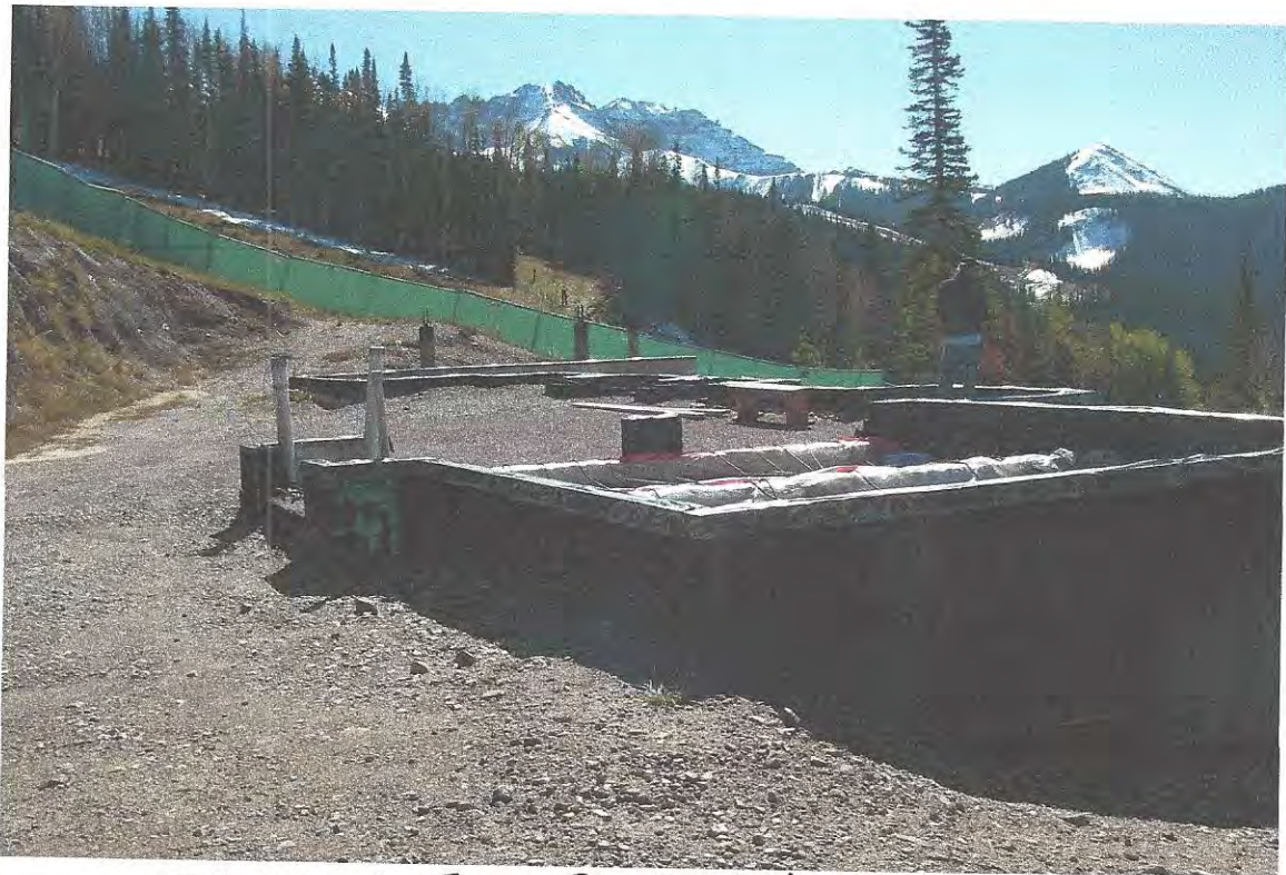
EXISTING FOUNDATION & AUTO COURT
