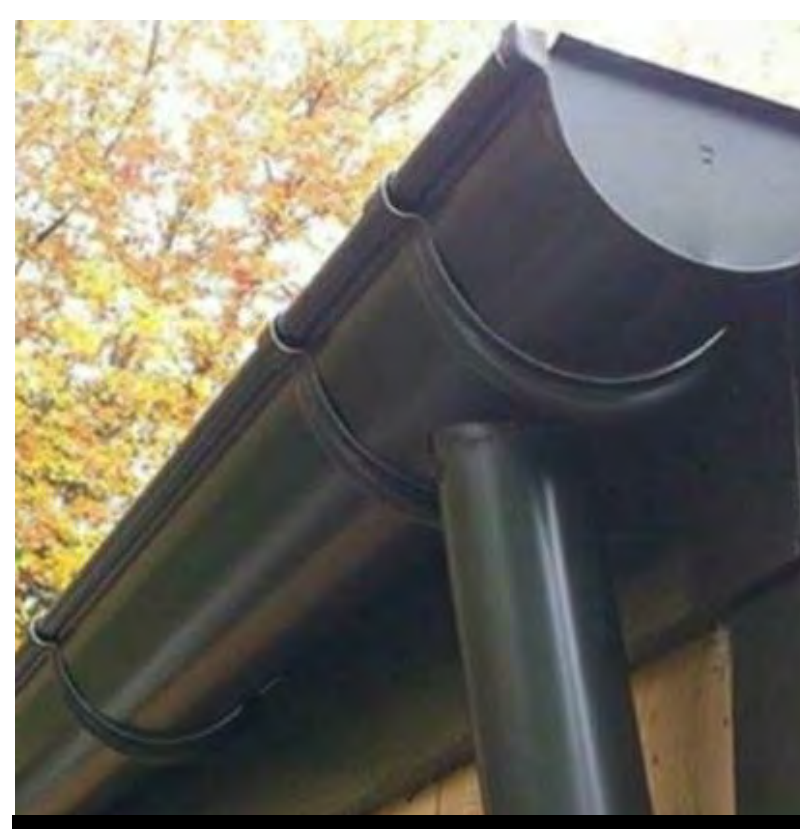
GUTTER - BLACK 1/2" ROUND ALUMINUM GUTTERS WITH METAL MESH LEAF GUARDS, ATTACHED TO 4" ROUND ALUMINUM DOWNSPOUTS. BLACK TO MATCH ROOF. HEAT TRACE WHERE NEEDED
