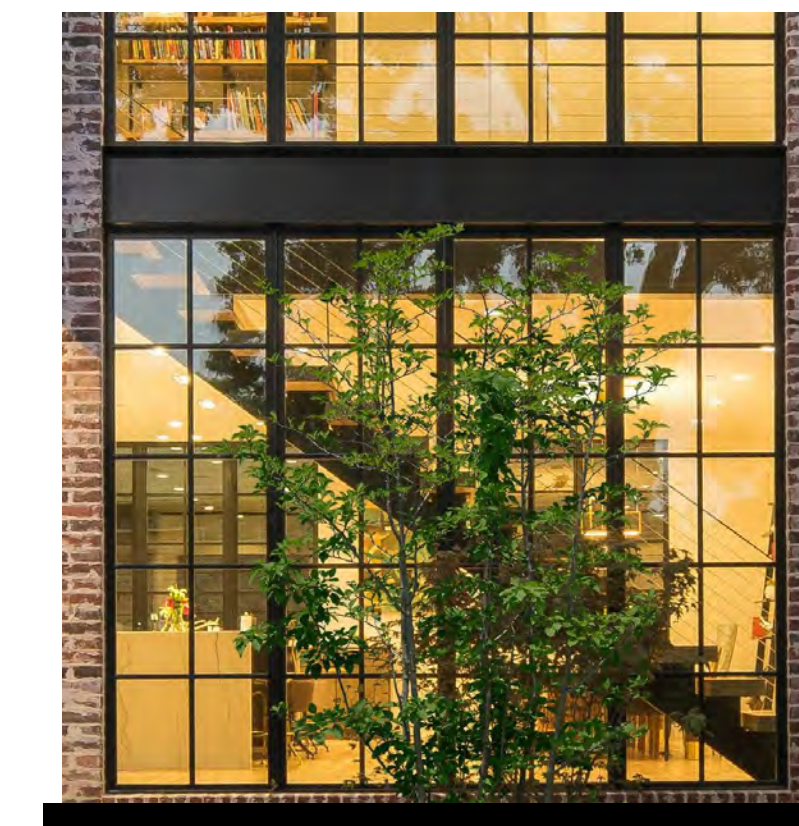
WINDOWS - BLACK ALUMINUM CLAD WOOD WINDOWS, BLACK TO MATCH ROOF, GUTTERS AND DOORS
