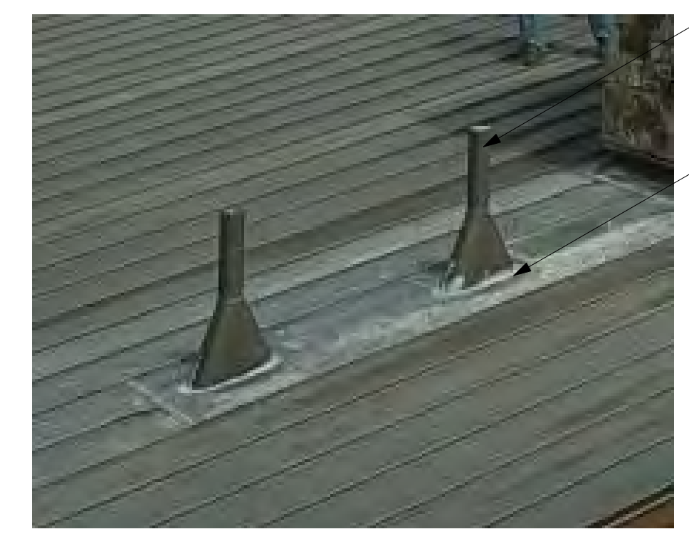
4 FLASHING @ PLUMBING VENTS 3" = 1'-0"
