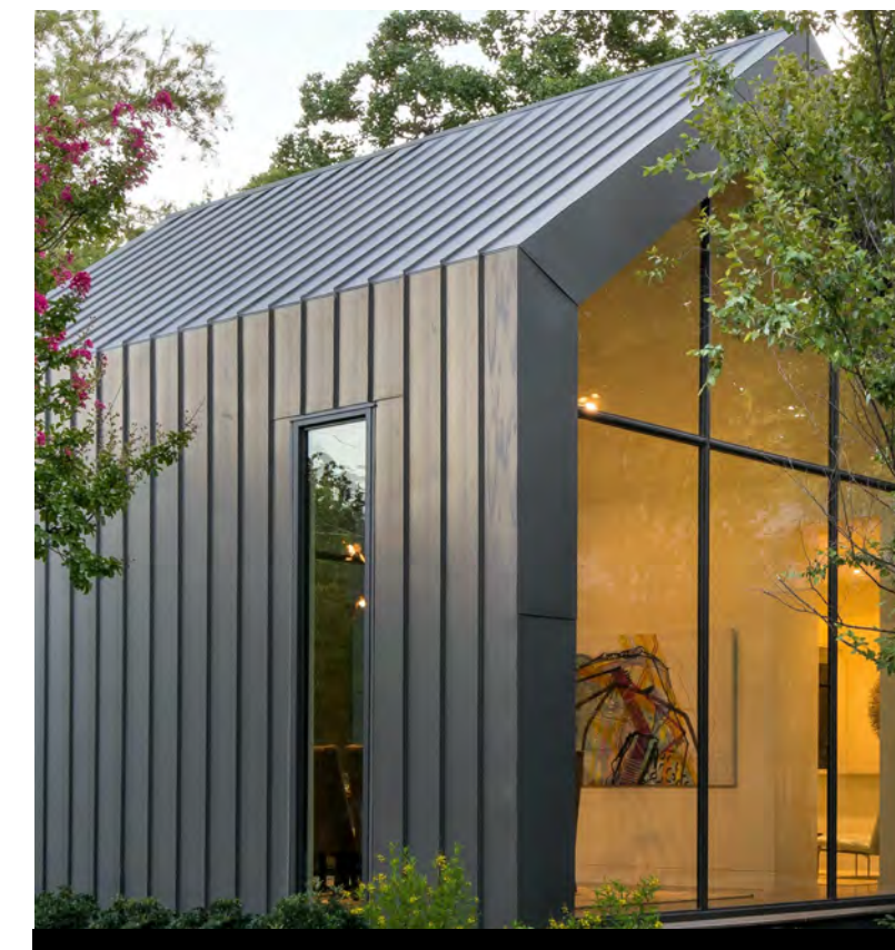
METAL SIDING - BLACK STANDING SEAM METAL SIDING 16" O.C. RUN IN A VERTICAL PATTERN
