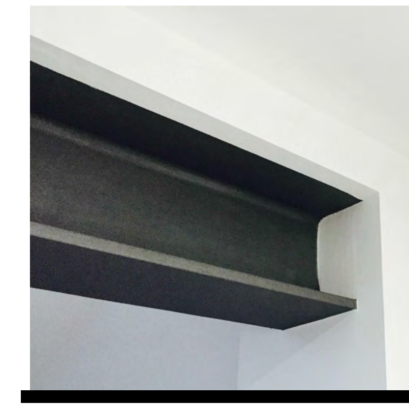
EXPOSED METAL - BLACK WH OR C CHANNEL BEAMS AND 3/16 BENT PLATE STEEL IN PENETROL PATINA FINISH OR PAINTED BLACK TO MATCH ROOF, WINDOWS AND DOORS
