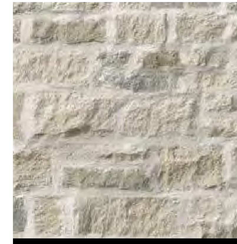
STONE ROUGH (R) - LIMESTONE STONE BASE: ROUGH CUT LIMESTONE IN VARYING SIZES FROM 6"-14" IN HEIGHT AND 10"-24" WIDE. NEUTRAL WARM WHITE AND LIGHT GREY COLOR TONS. LAID IN HORIZONTAL RANDOM STACK WITH AN OVER GROUT TECHNIQUE IN WHITE
