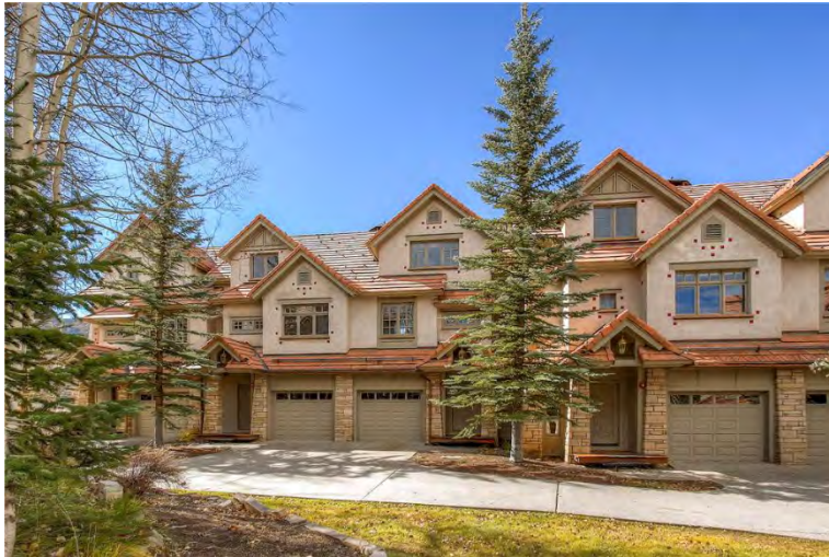
Aspen Ridge Condominiums (Estimated +/- 45% Stucco on the primary street façade)
