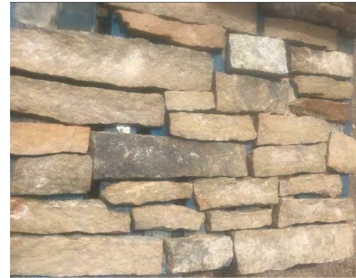
STONE VENEER TELLURIDE STONE COMPANY COLOR - SAGE LEDGESTONE (DRY STACKED)
