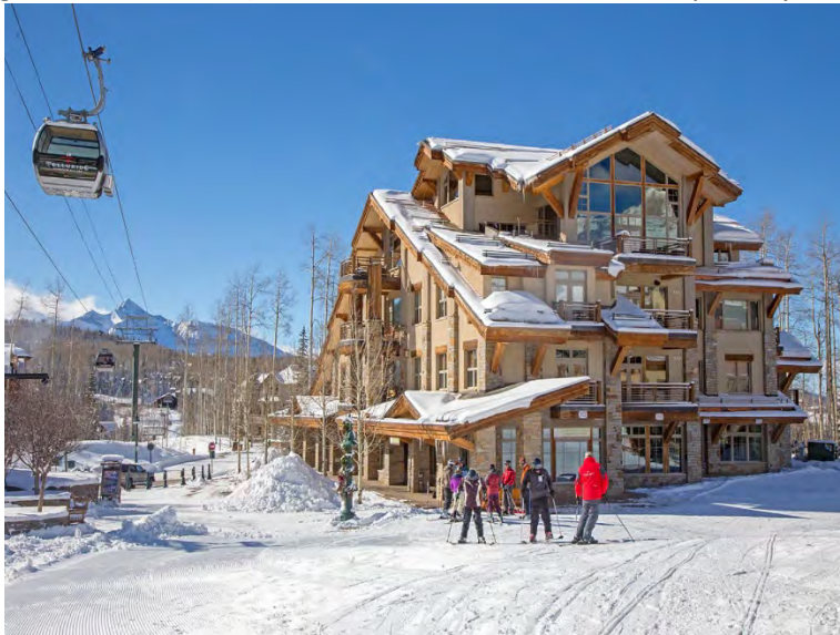
Granita (Village Center - Estimated +/- 50% Stucco)
