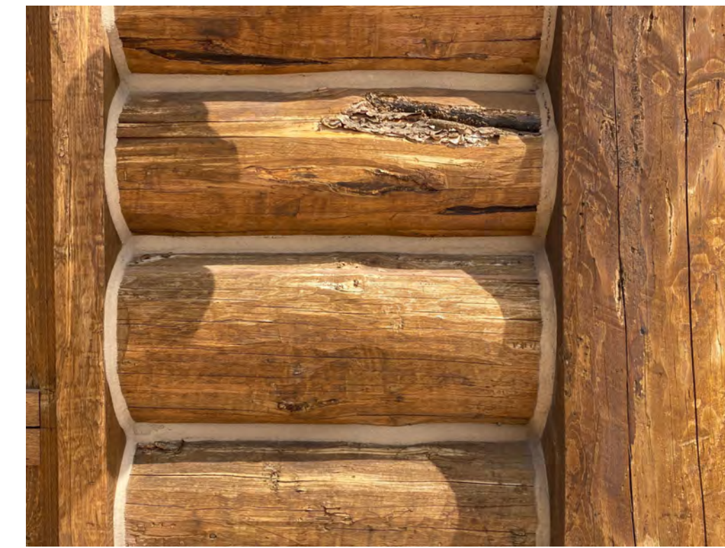
Hand peeled log siding with log post corners and chinking
