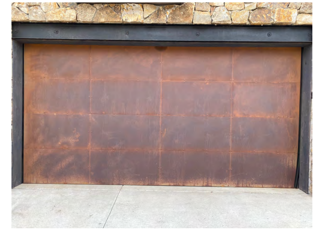
Garage door rusted metal flat 2'x4'
