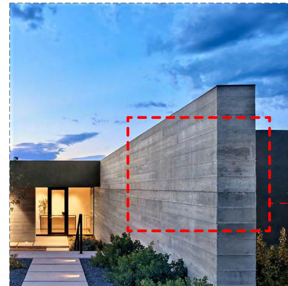
BOARD FORMED CONCRETE
