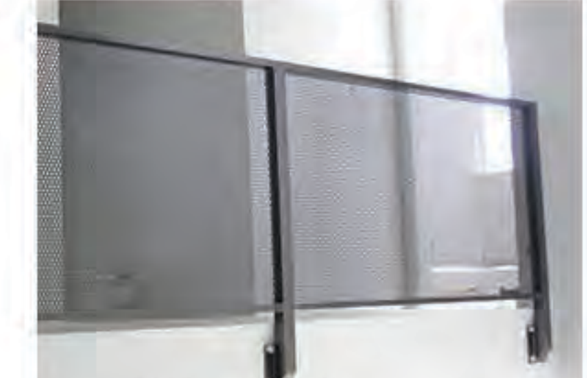
METAL RAILING BLUING OIL FINISH
