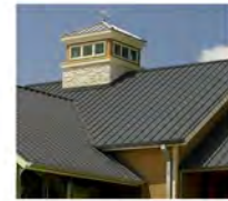
2" SNAP LOCK STANDING SEAM MTL ROOFING FINISH: MUSKET GRAY MANUFACTURER: DREXTEL METALS
