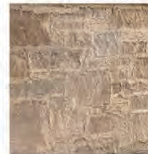
6" STONE VENEER WITH MINER'S SHMEAR GROUT JOINTS
