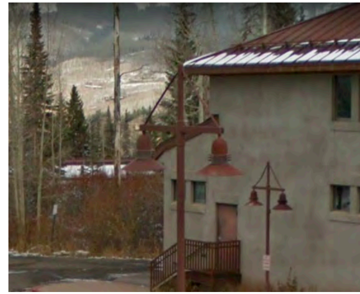
Existing Exterior Light Fixture
