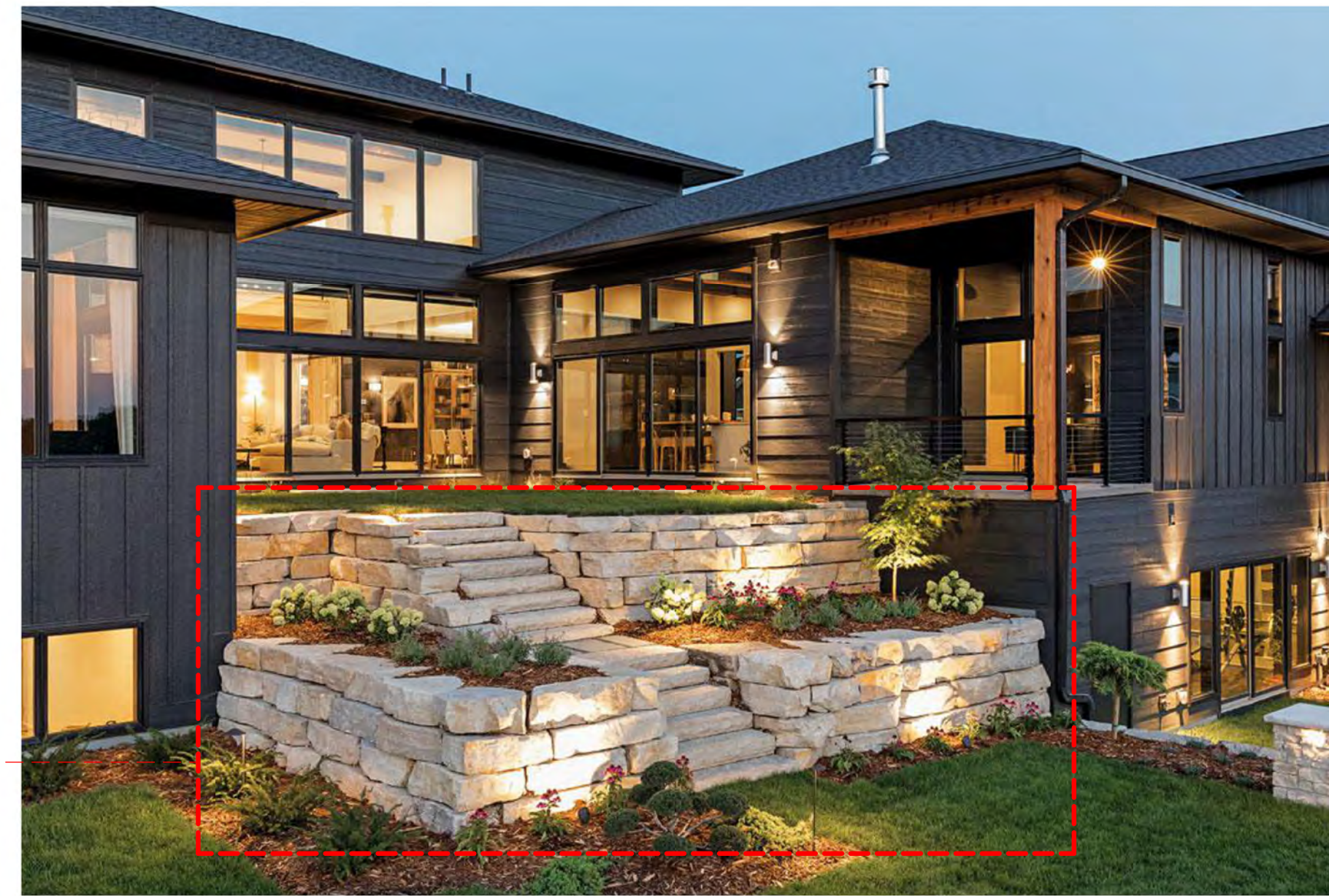
STONE RETAINING WALL
