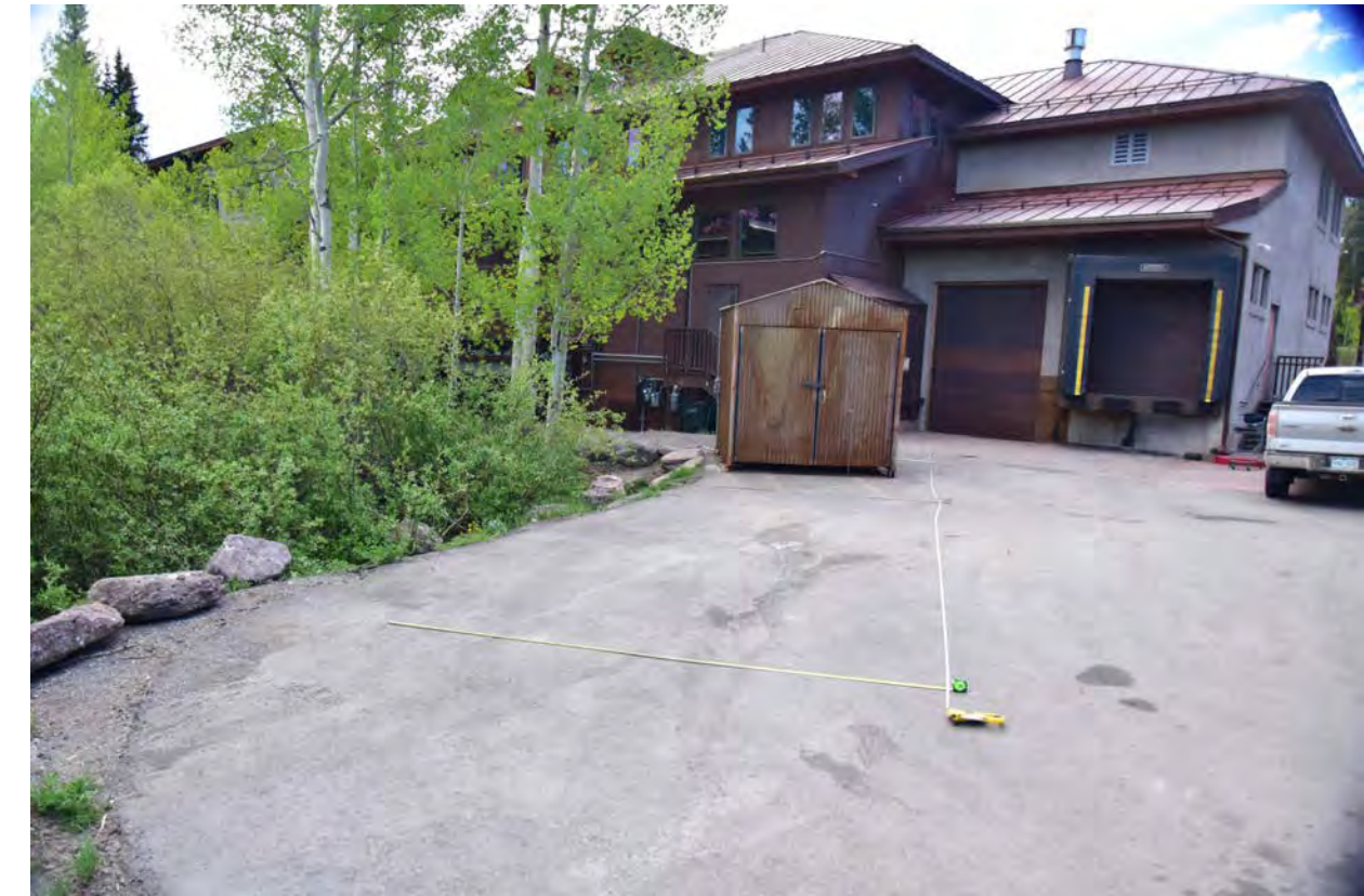
EXISTING TRASH AND LOADING AREA
