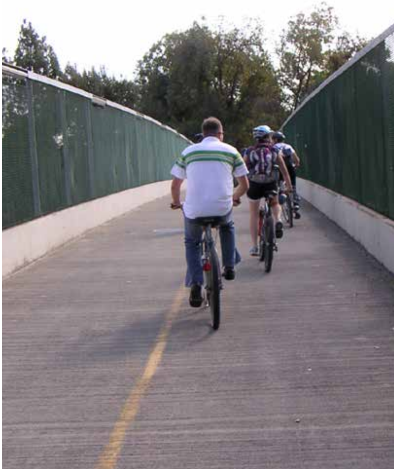
Overcrossings provide connections over barriers where at-grade crossings are infeasible or undesired.
