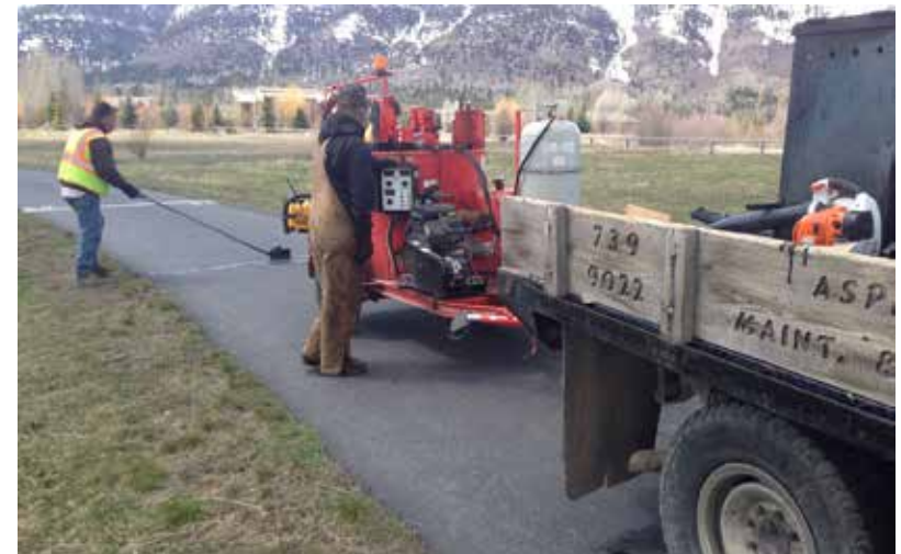
Crack sealing operations help to extend that lifespan of asphalt trails.
