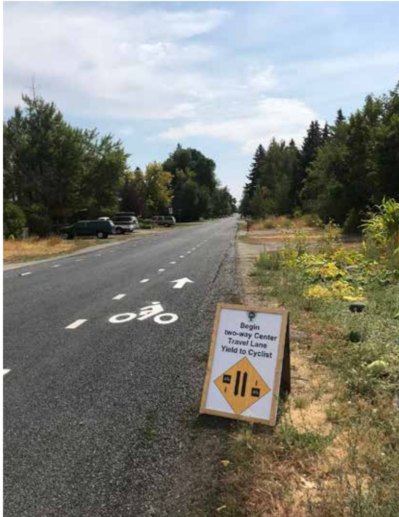
Advisory shoulders prioritize shoulder space for pedestrians and bicyclists on narrow roads. Image credit: Michael David.
