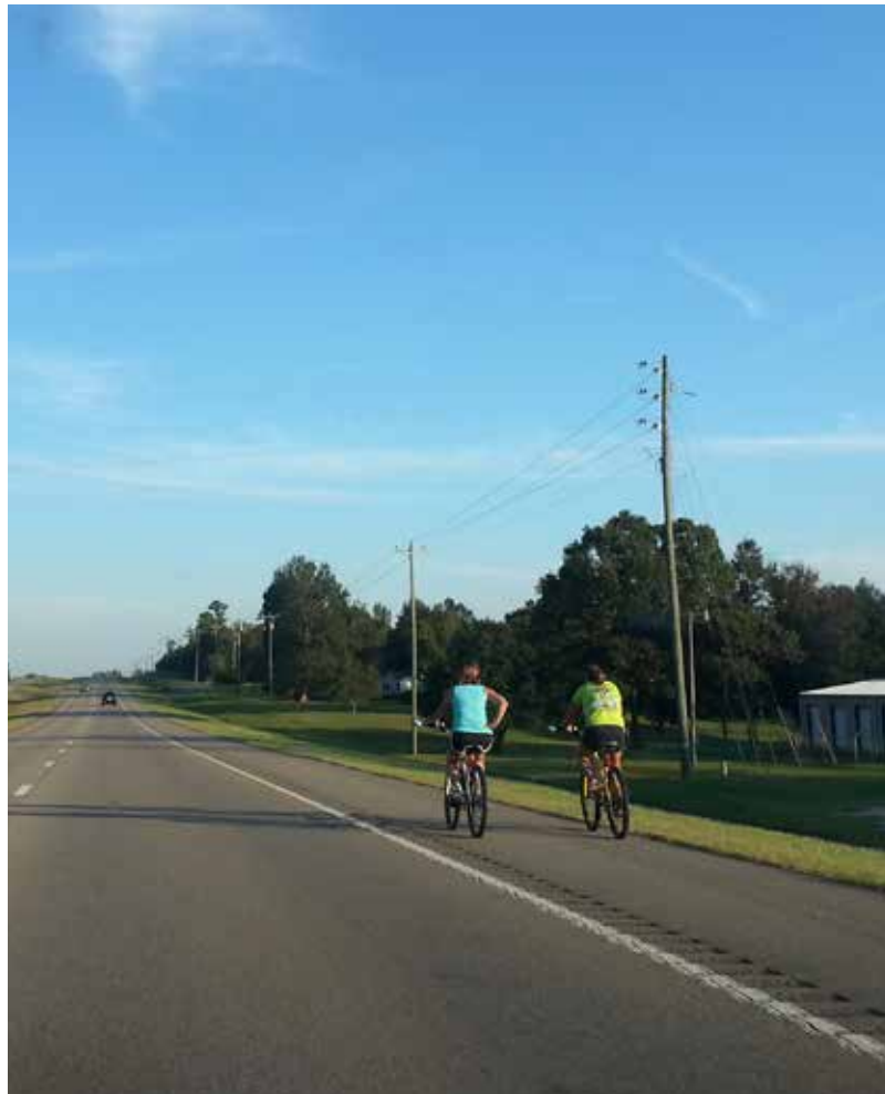
Wide paved shoulders provide pedestrians and bicyclists with usable space outside of the vehicle travel lane.
