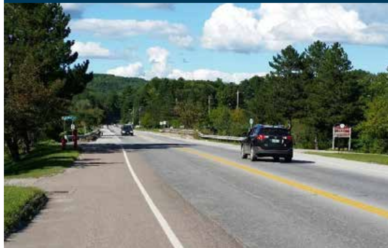
Wide paved shoulders provide pedestrians and bicyclists with usable space outside of the vehicle travel lane.
