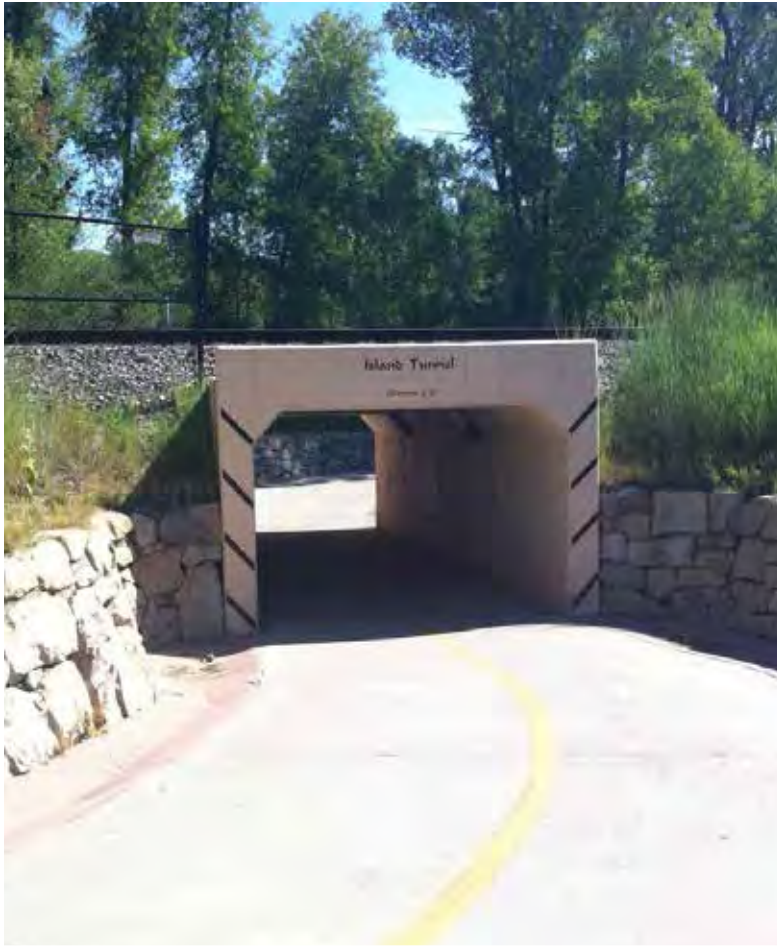
Undercrossings provide connections over barriers where at-grade crossings are infeasible or undesired.
