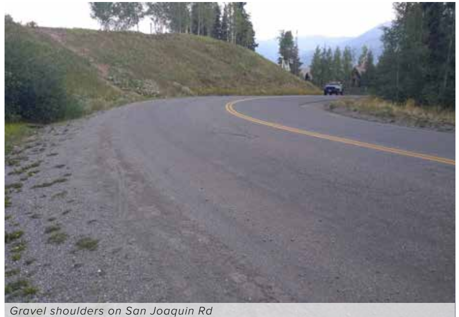
Gravel shoulders on San Joaquin Rd
