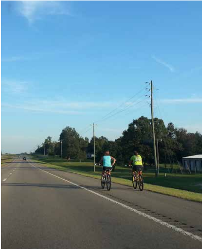
Wide paved shoulders provide pedestrians and bicyclists with usable space outside of the vehicle travel lane.
