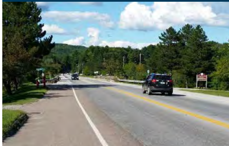
Wide paved shoulders provide pedestrians and bicyclists with usable space outside of the vehicle travel lane.
