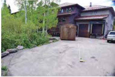
EXISTING TRASH AND LOADING AREA
