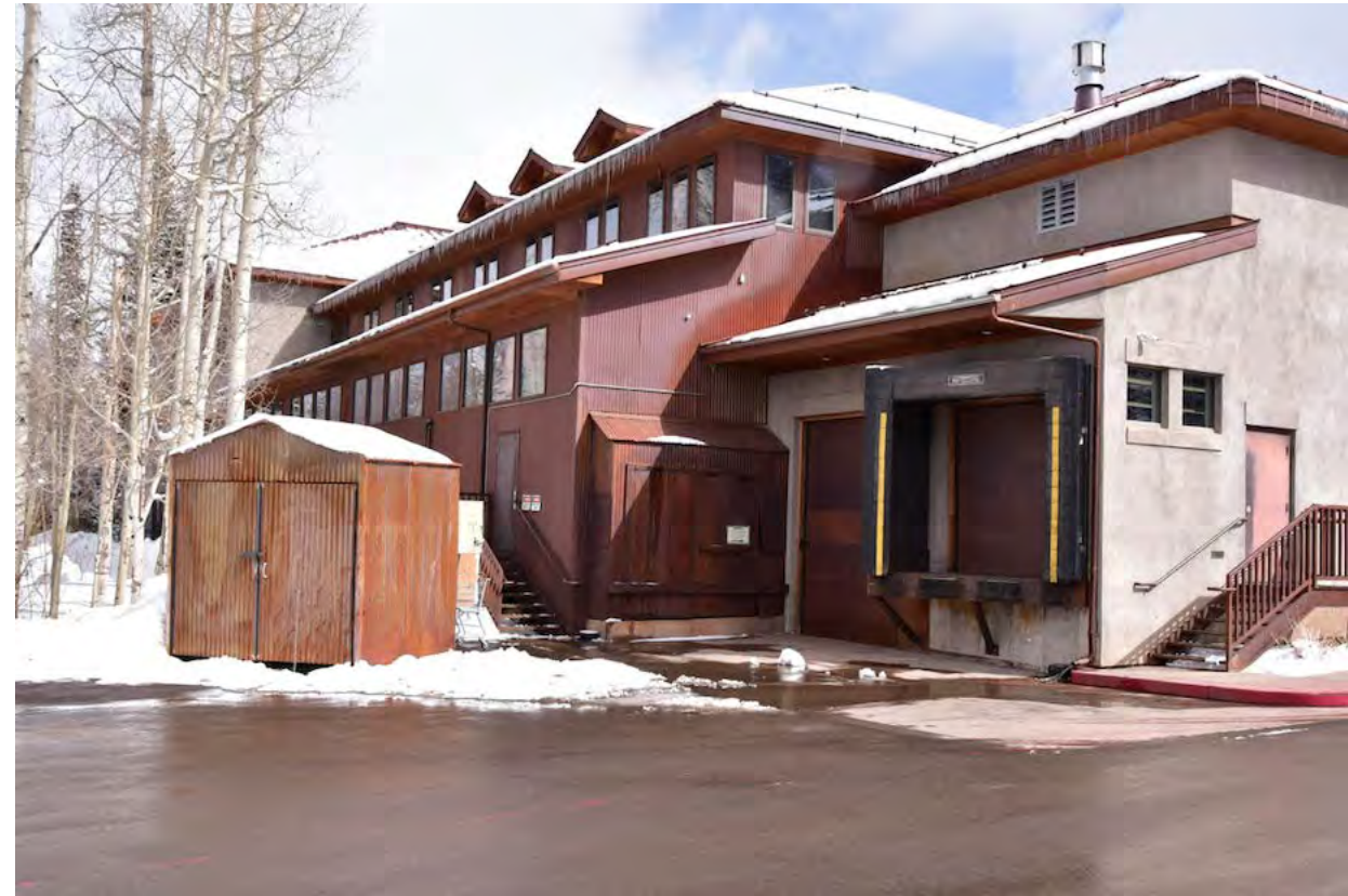
EXISTING SITE PIC 4
