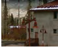
Existing Exterior Light Fixture
