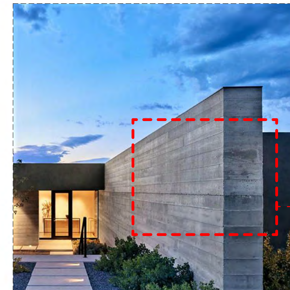
BOARD FORMED CONCRETE
