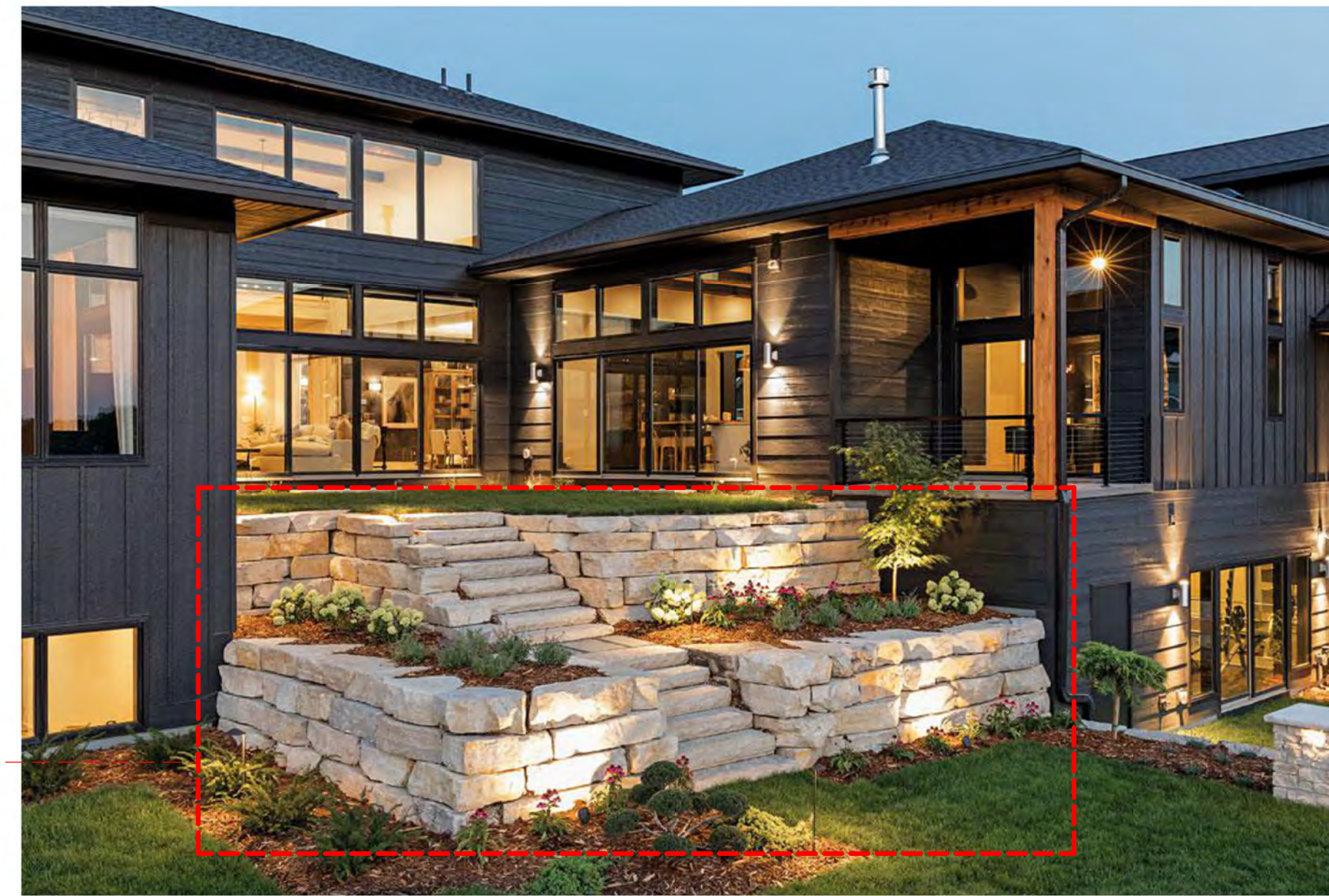
STONE RETAINING WALL
