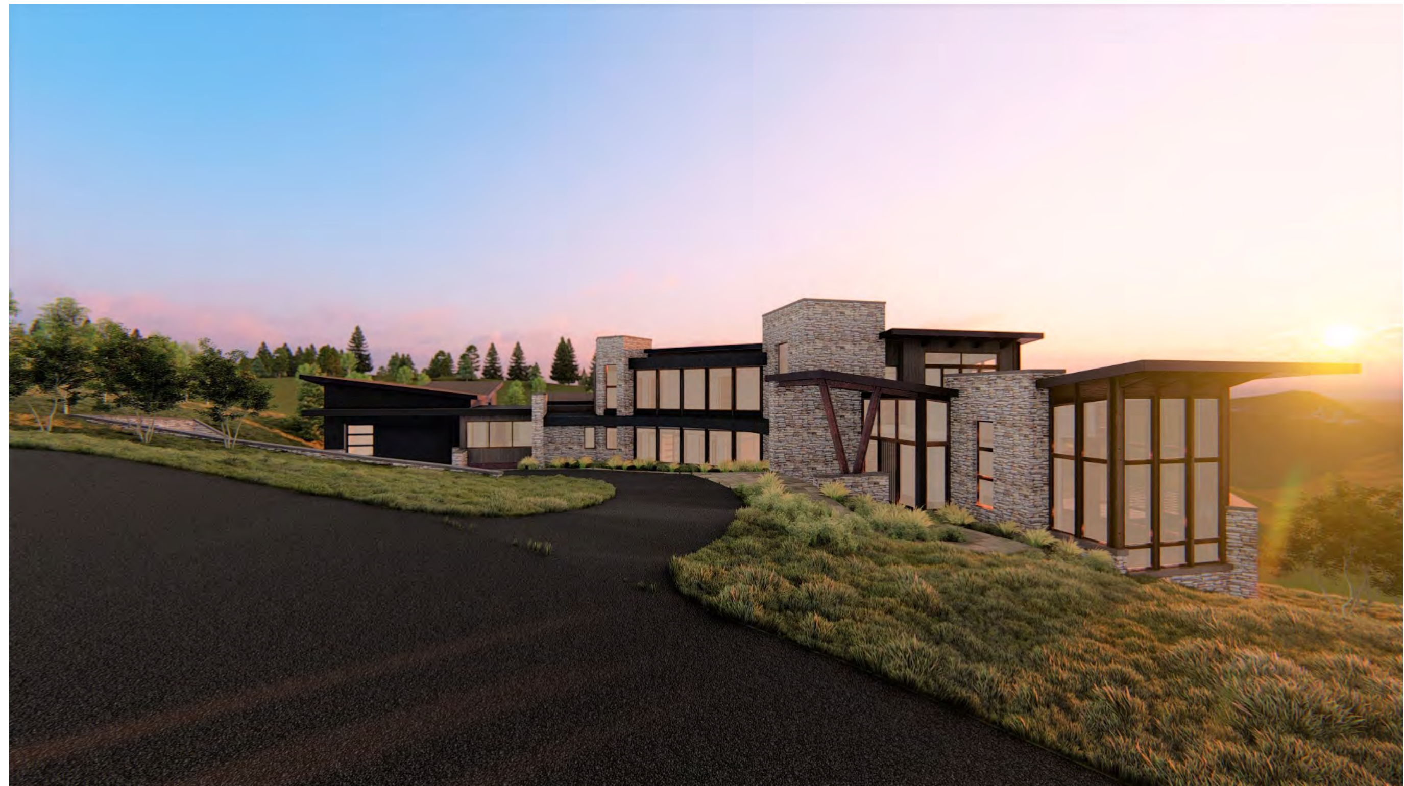
G.E. ENCROACHMENT AS SEEN FROM PENNINGTON PLACE
