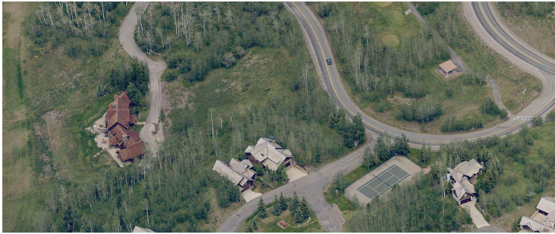
3 AERIAL WEST PHOTO 12" 1'-0"
