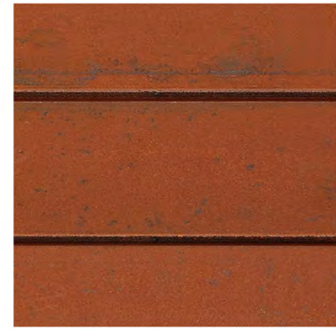
RUSTED HORIZONTAL STEEL SIDING
