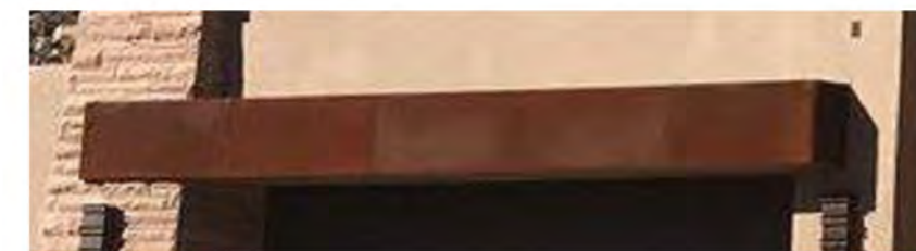
RUSTED STEEL FASCIA & SOFFIT
