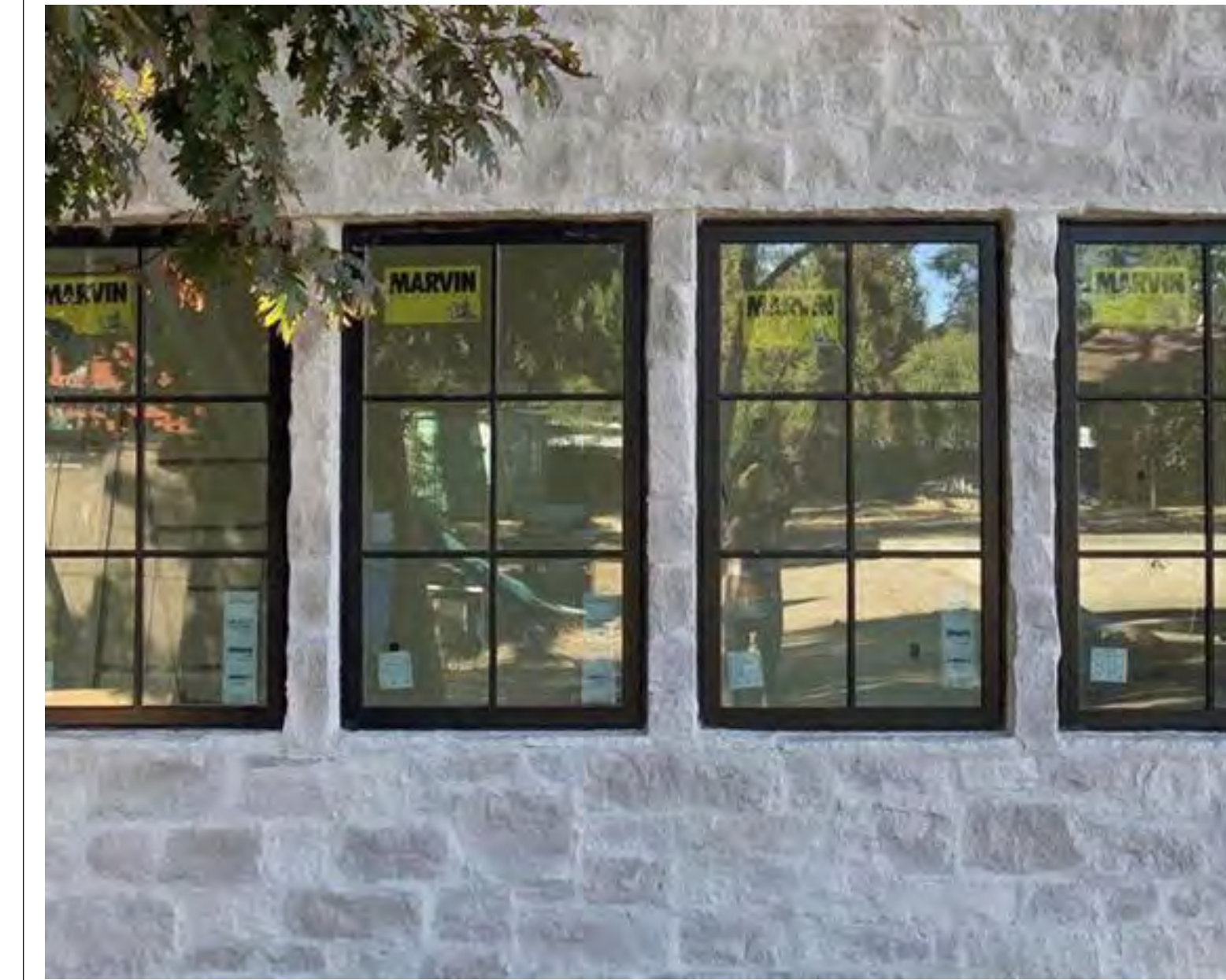
STONE LAY UP - OVER GROUT (BITTERED)
