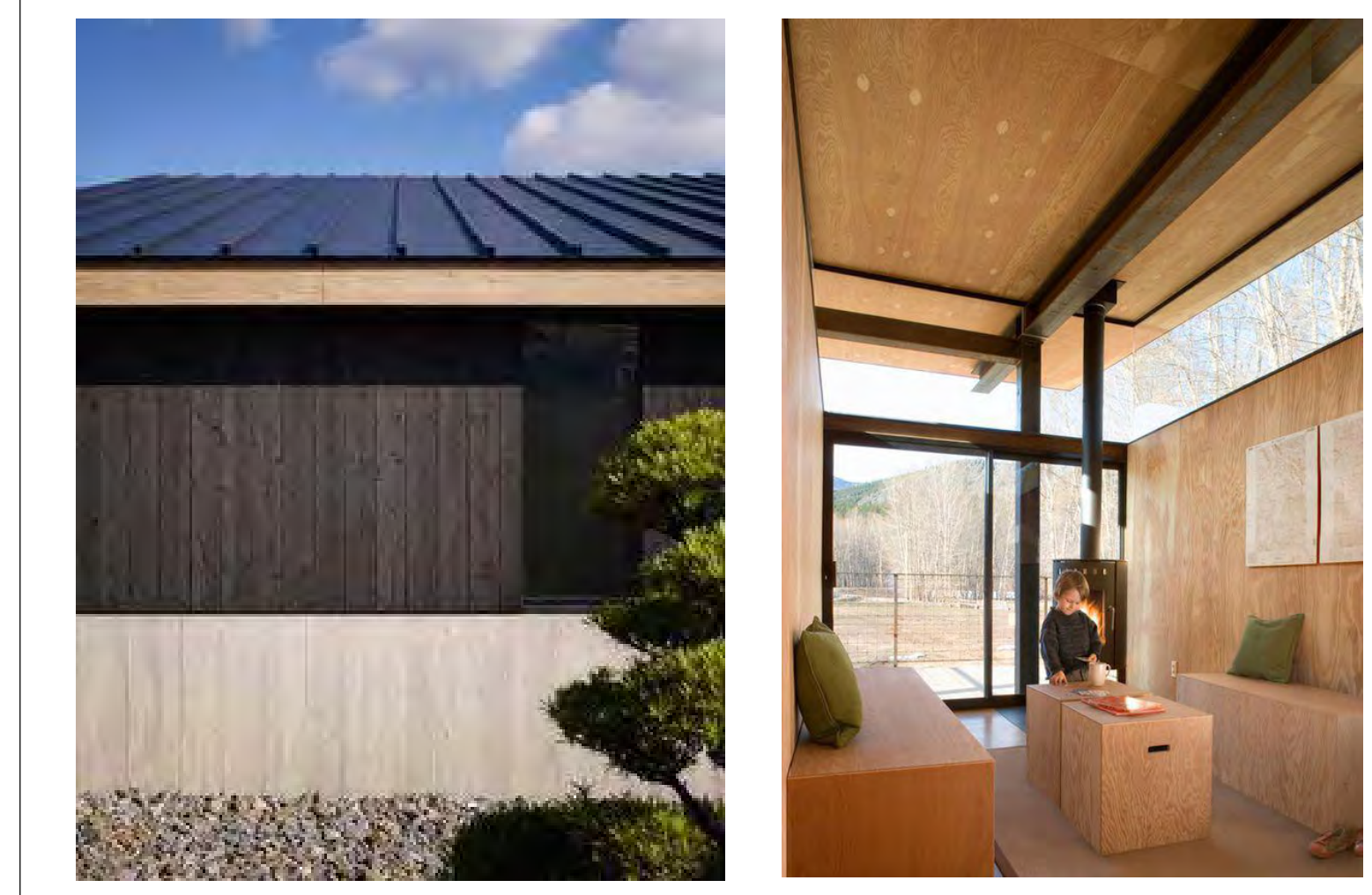
STANDING SEAM METAL ROOF EXPOSED STEEL STRUCTURE
