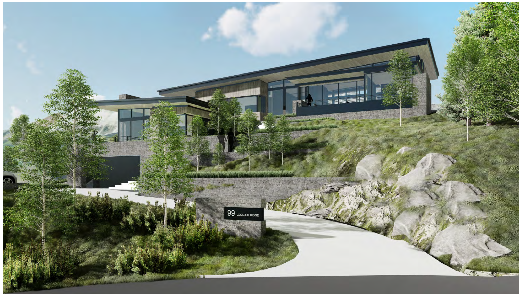
1) FROM THE ENTRY DRIVE AT THE JUNCTION OF MOUNTAIN VILLAGE BOULEVARD AND LOOKOUT RIDGE DRIVE. THE STRUCTURED BOULDER WALL IS MEANT TO BREAK DOWN VERTICAL SCALE OF NECESSARY RETAINAGE FOR A SAFE DRIVEWAY IN CONGRUENCE WITH THE LANGUAGE OF THE HILLSIDE.
