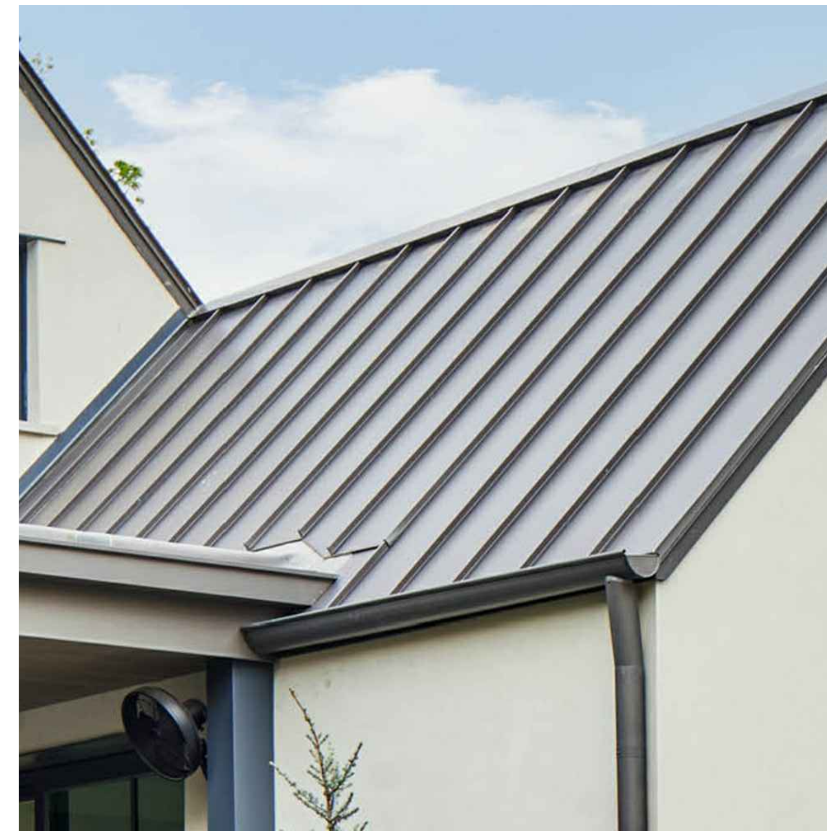
STANDING SEAM METAL ROOF
