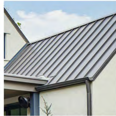
STANDING SEAM METAL ROOF
