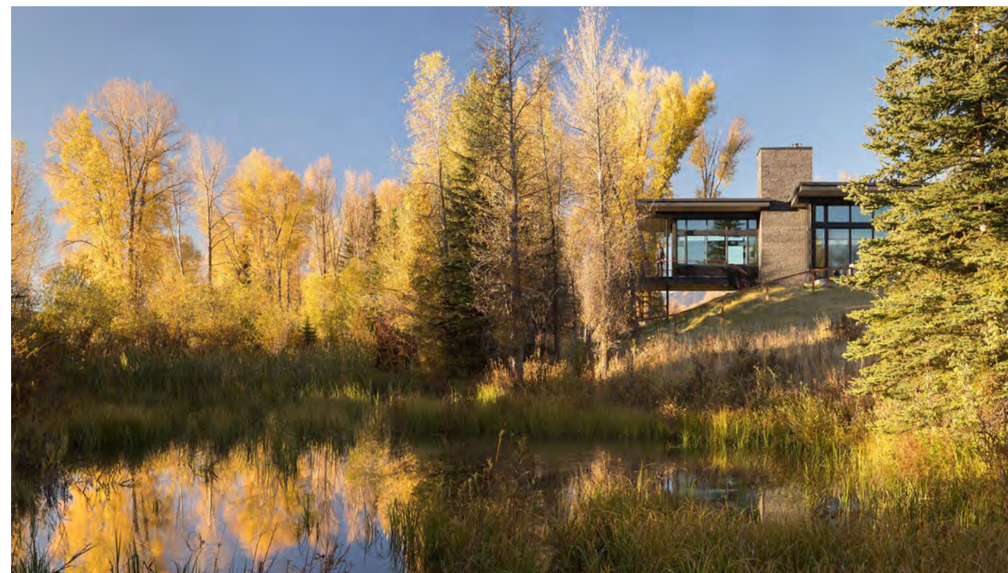
DARK PREFINISHED ALUMINUM SHEET METAL AT WINDOWS & FASCIAS MATTE FINISH (NON REFLECTIVE)
