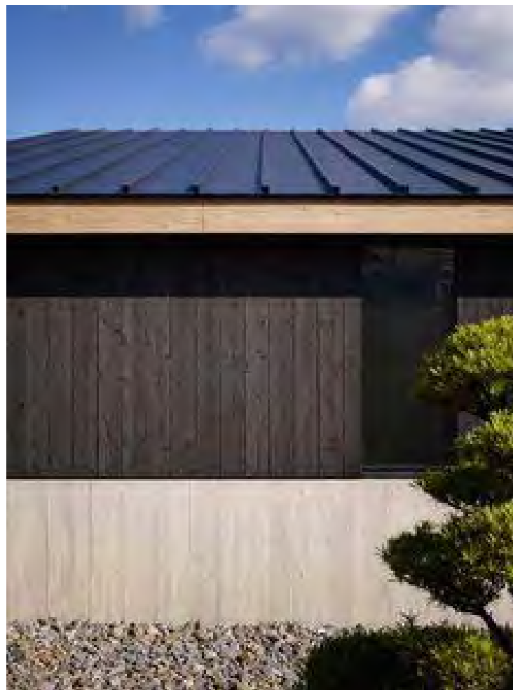
STANDING SEAM METAL ROOF
