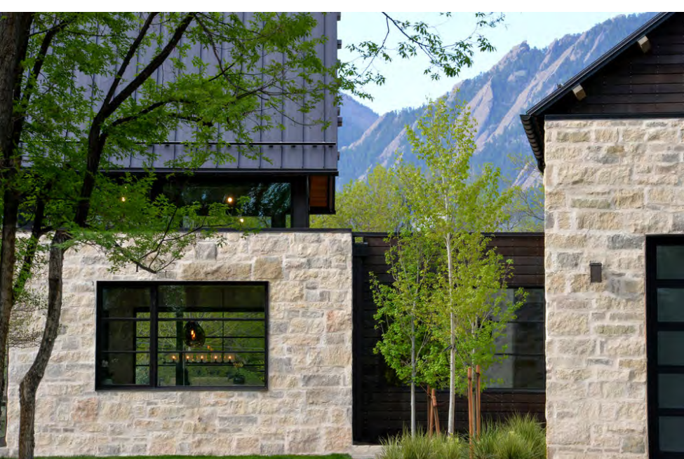
STONE BASE - BUTTERED GROUT APPLICATION
