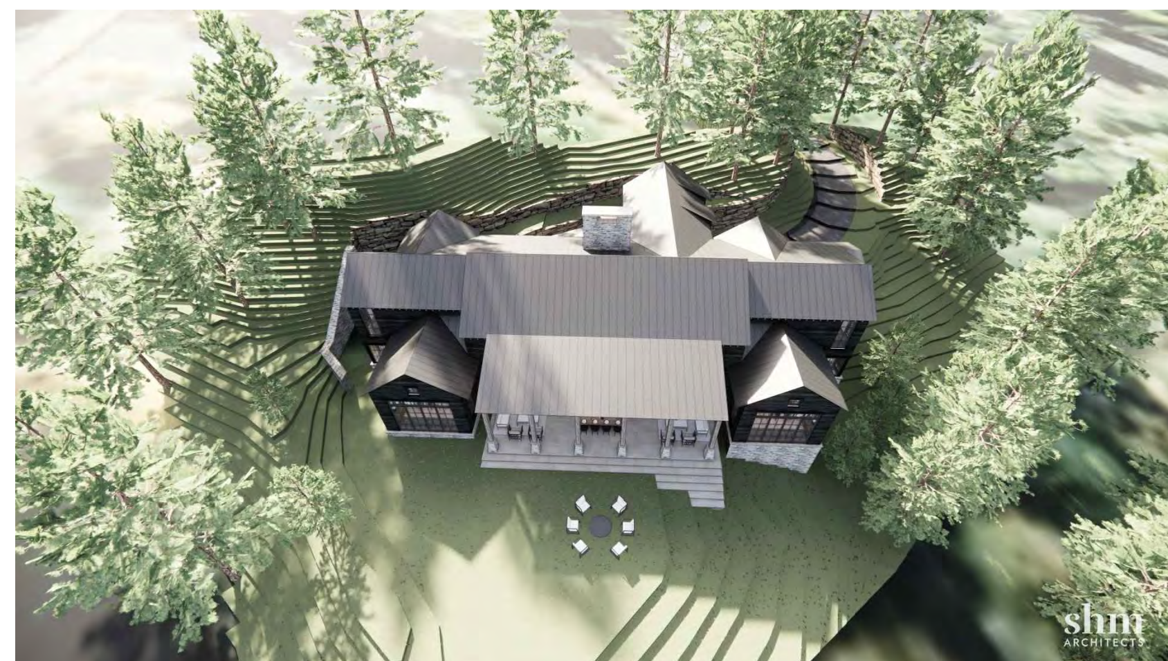
OVERVIEW LOOKING SOUTH
