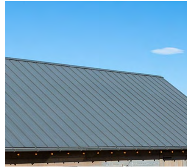
Roofing / (Drip Edge) - Standing Seam 16" O.C.
