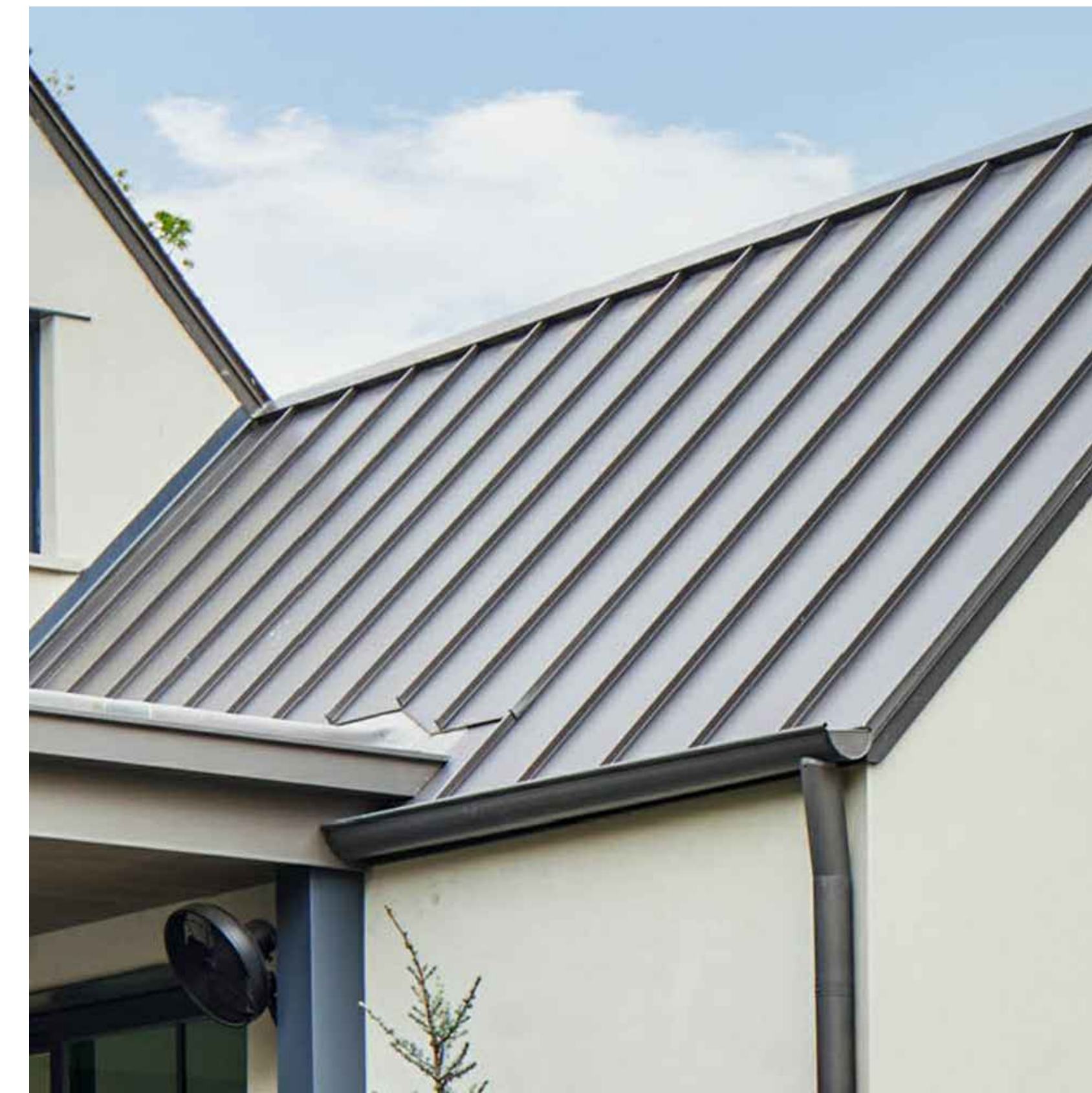
STANDING SEAM METAL ROOF 24 GAUGE
