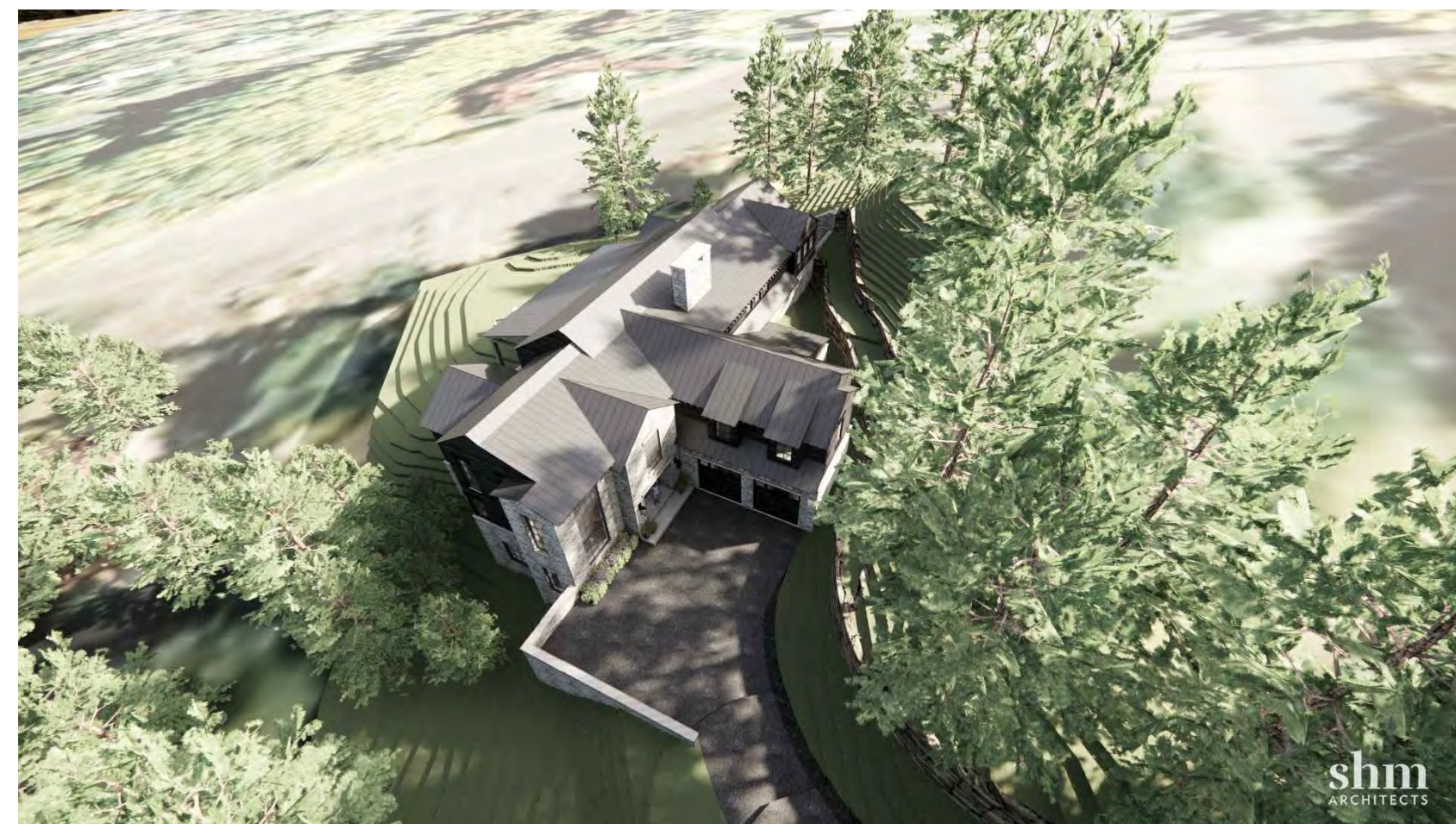
OVERVIEW LOOKING NORTH EAST
