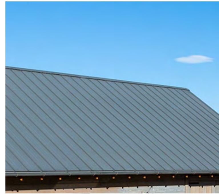
Roofing / (Drip Edge) - Standing Seam 16" O.C.
