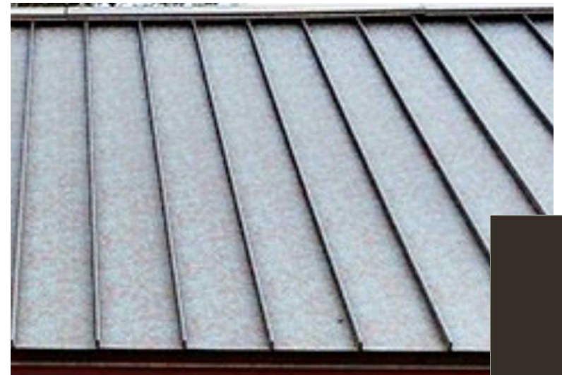
PRIMARY ROOF SNAP-LOCK STANDING SEAM
