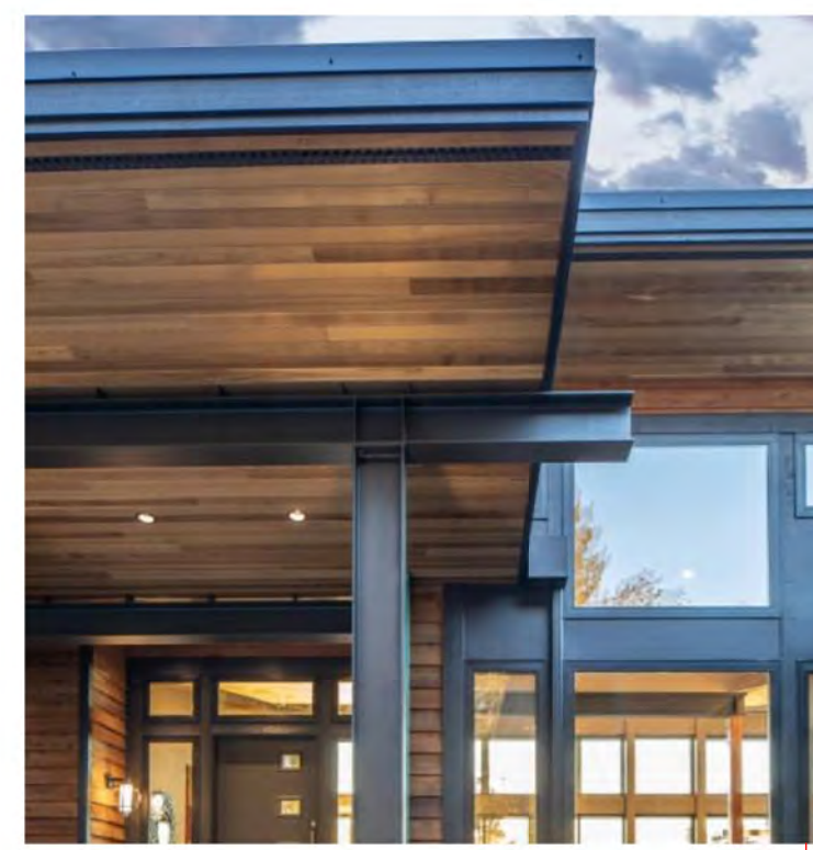
STEEL STRUCTURE: EXPOSED WIDE FLANGE STEEL, DARKING BLUING FINISH OR OIL RUB
