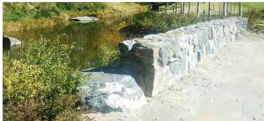
1 Stone Bridge Reference Imagery Not to scale NOTE: The image is a Sample/Reference of the design intent, the stone veneer will be similar to the building veneer but be a more rustic/rugged interpretation as
