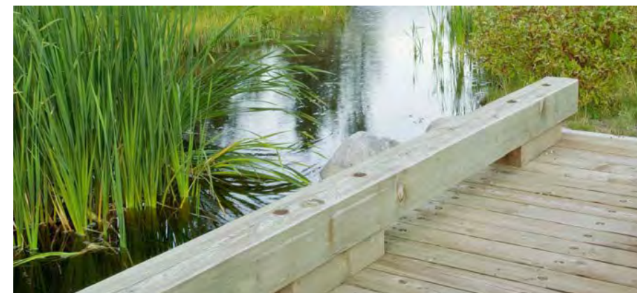
2 Wood Bridge Reference Imagery Not to scale NOTE: The image is a Sample/Reference of the design intent, the wood curb is included as a low barrier to prevent users from stepping off the edge.
