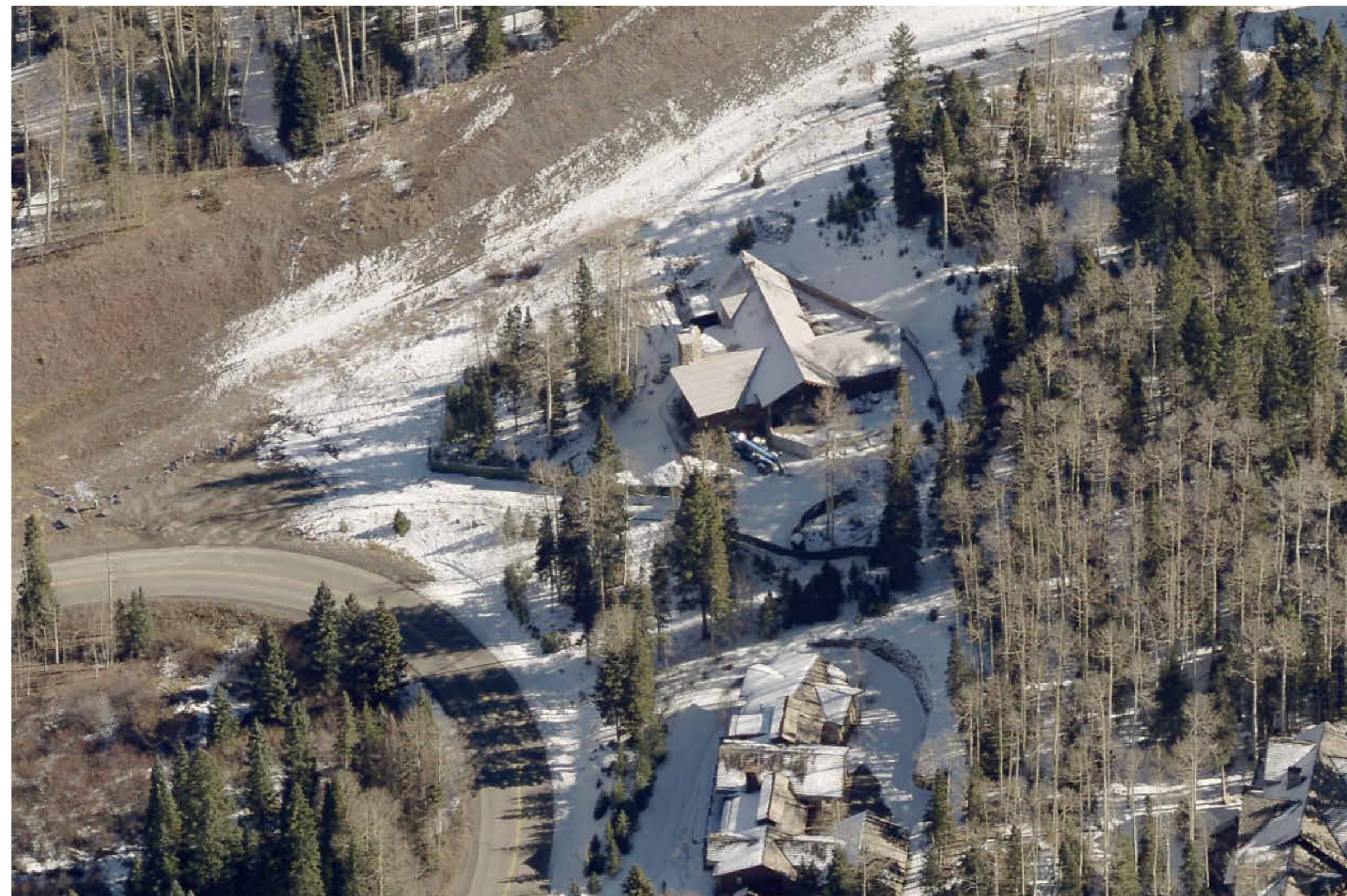
3 AERIAL WEST PHOTO 12" = 1'-0"
