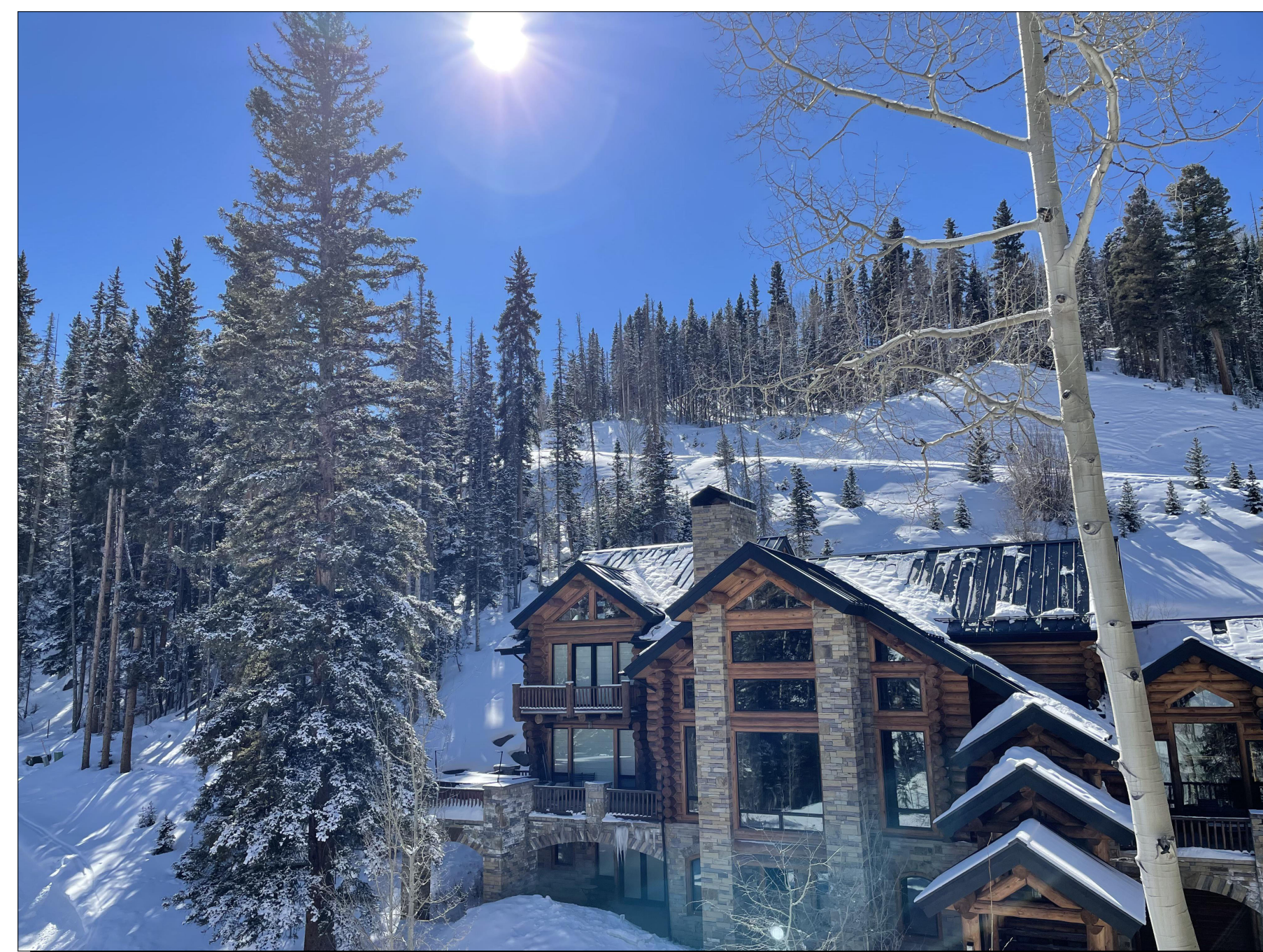
5_South View over Neighbor
