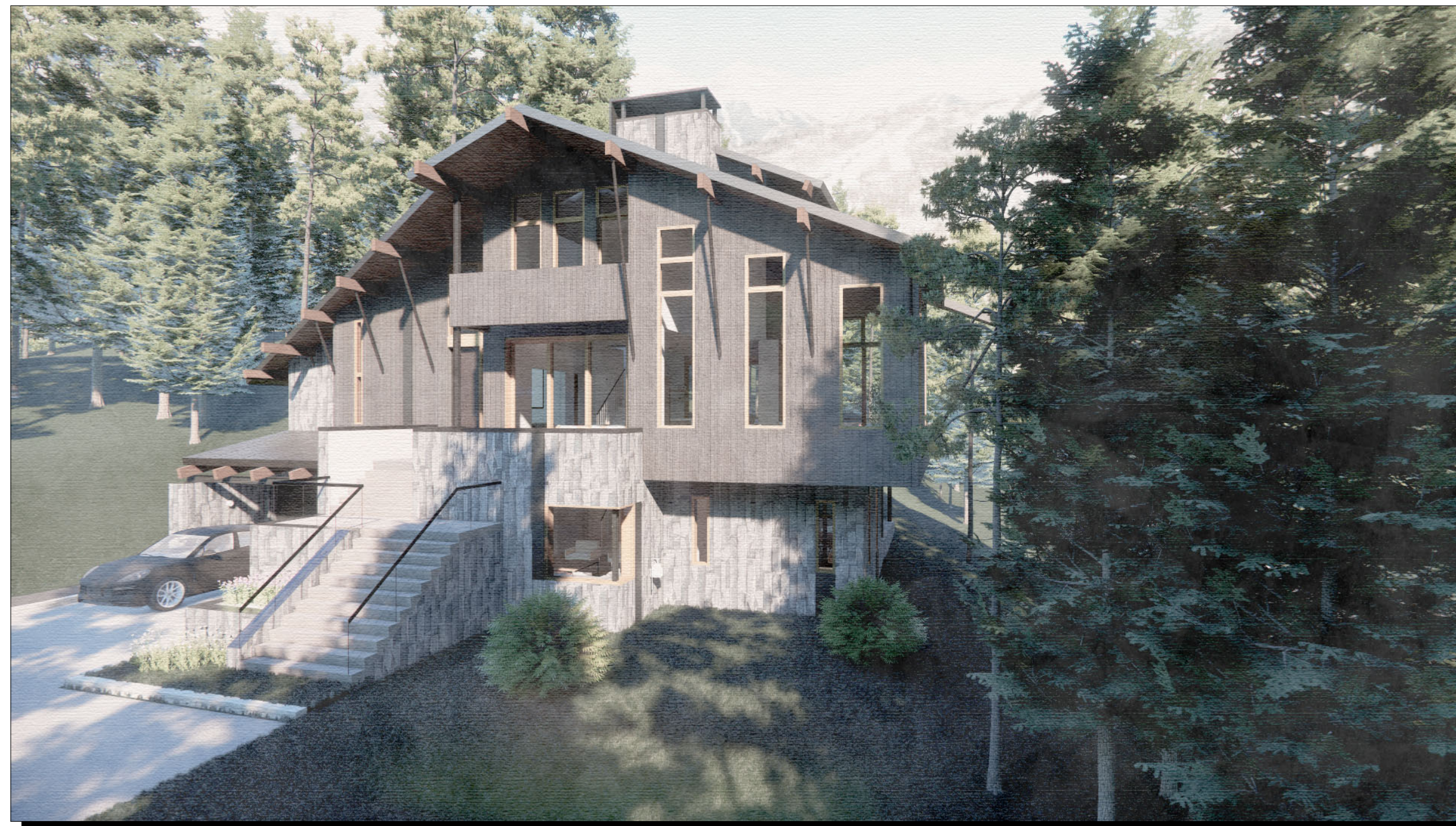
MAIN HOUSE SOUTH VIEW 1
